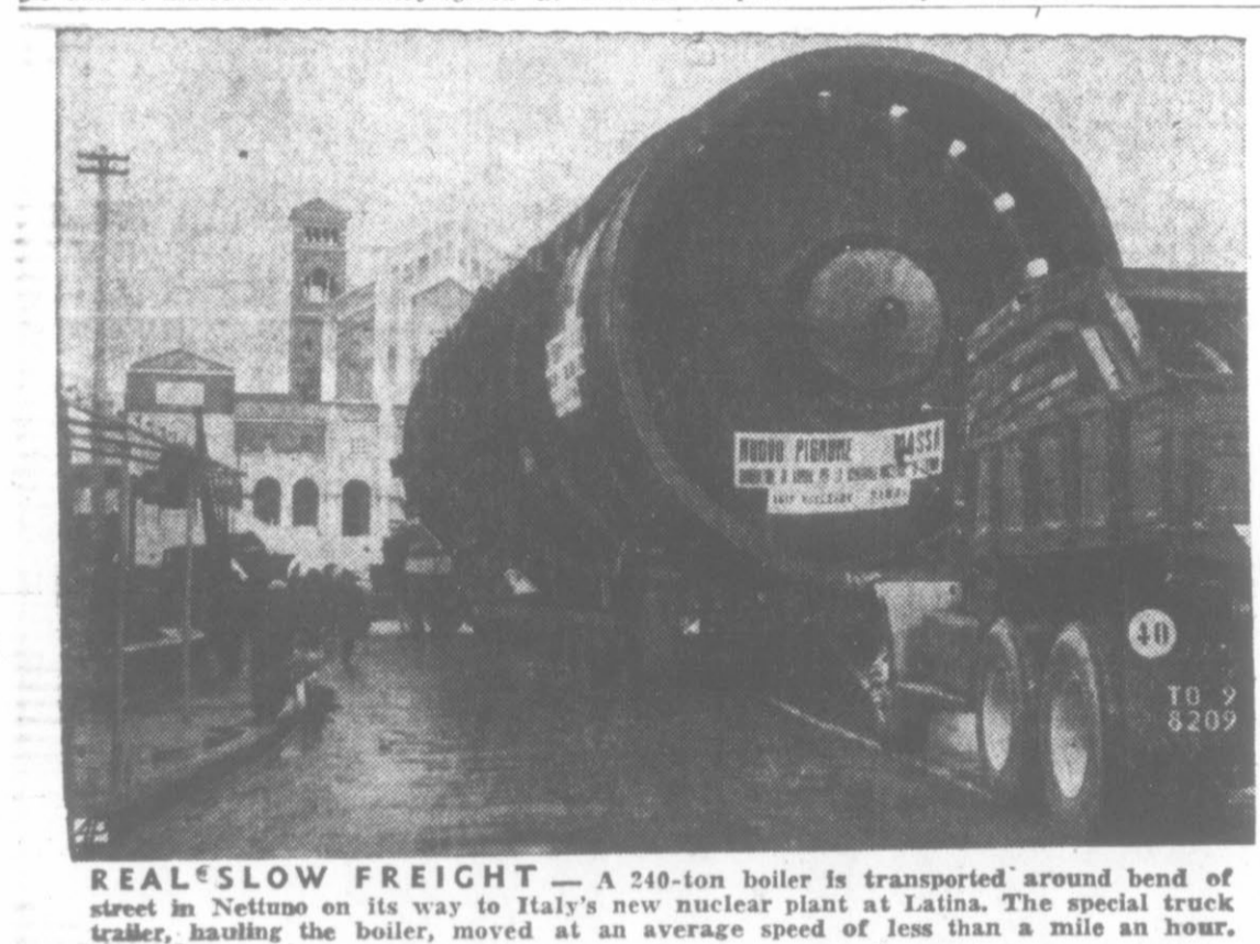
REAL SLOW FREIGHT — A 240-ton boiler is transported around bend of street in Nettuno on its way to Italy's new nuclear plant at Latina. The special truck trailer, hauling the boiler, moved at an average speed of less than a mile an hour.
