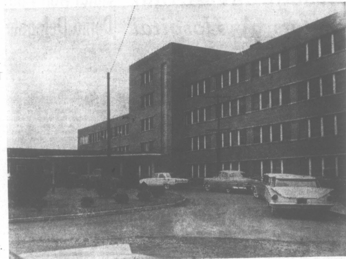
PITT MEMORIAL HOSPITAL . . . opened in 1951. Now another section is being built.
