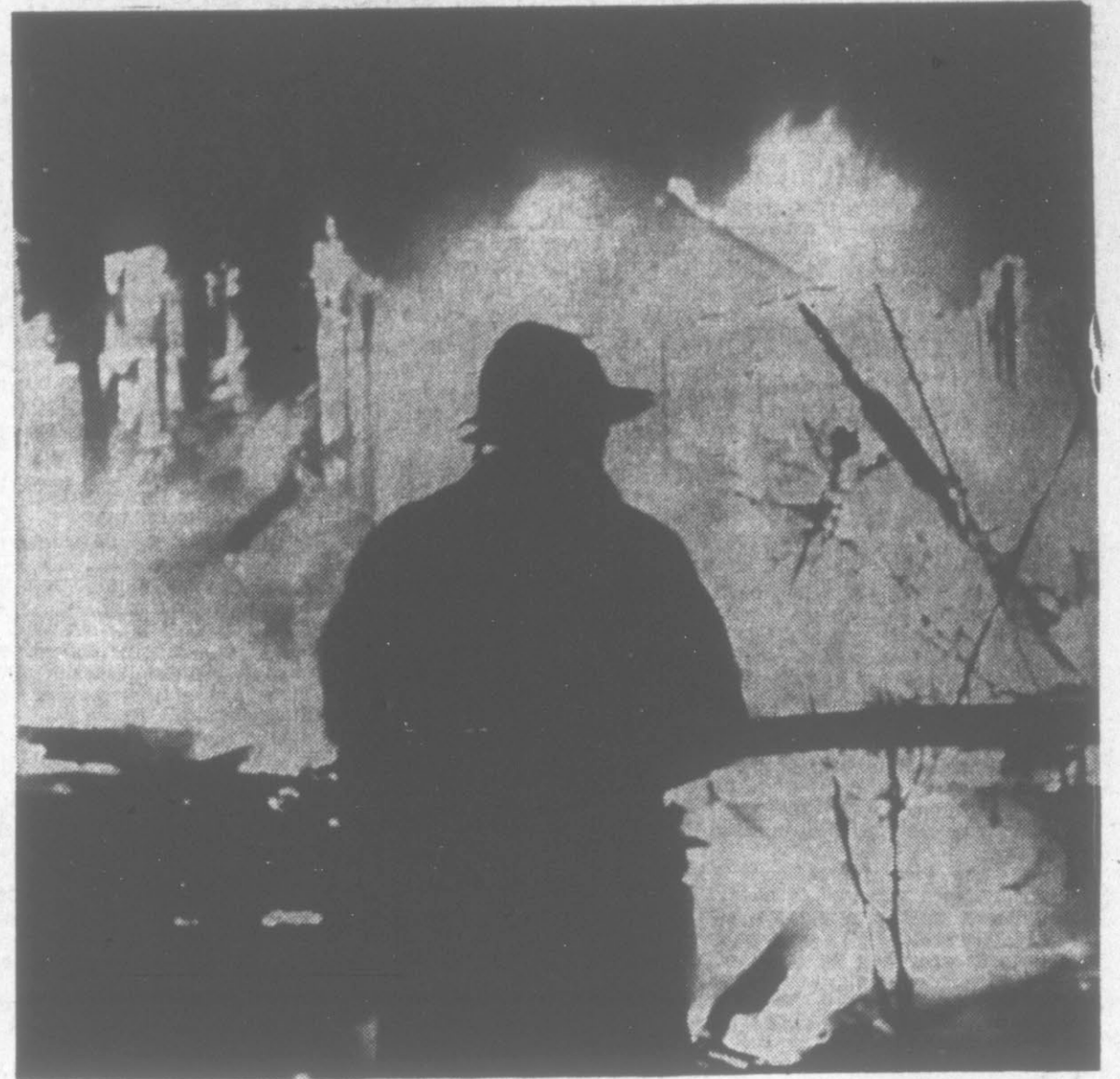
WATCH HOUSE BURN—Firemen from Lenoir and adjoining counties, after setting fire to an old dwelling north of Kinston many times last night in connection with a week-long fire school held there, stood by and watched the house burn to the ground following the night's schooling. Purpose of the house-burning was to demonstrate the effect of fog applications on the blaze. Sherman Pickard and Elwood Insko, instructors for the North Carolina Insurance Department, conducted the fire last night. Greenville Fire Department training officers Claude Christopher and Jenness Allen and volunteers Jimmy Smith and Stuart Savage participated in the class last night.
