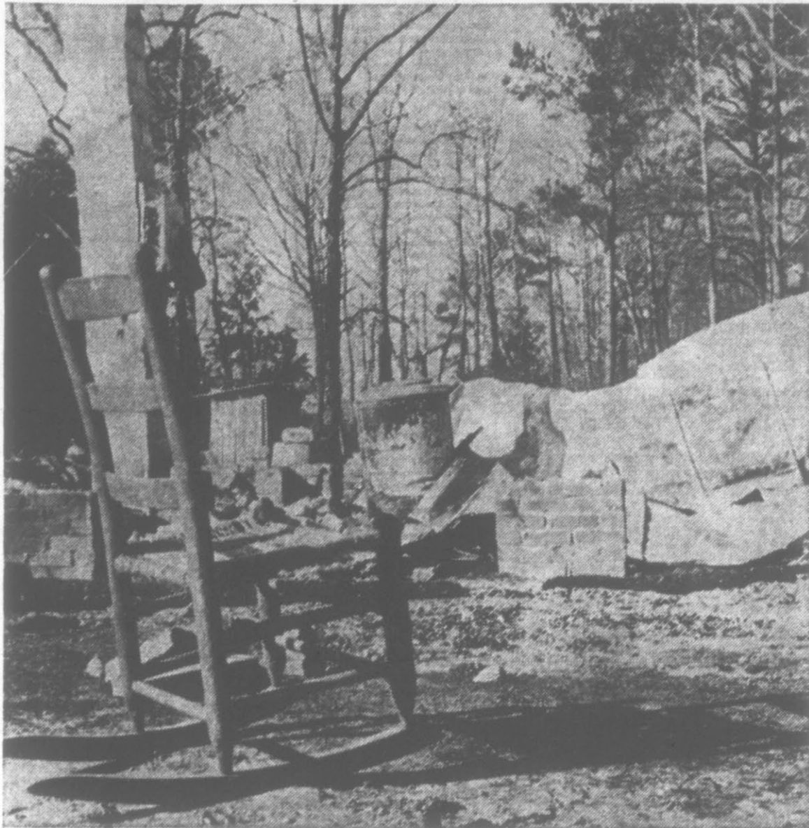
THE CHAIR . . . all that remains, in front of the destroyed dwelling.
