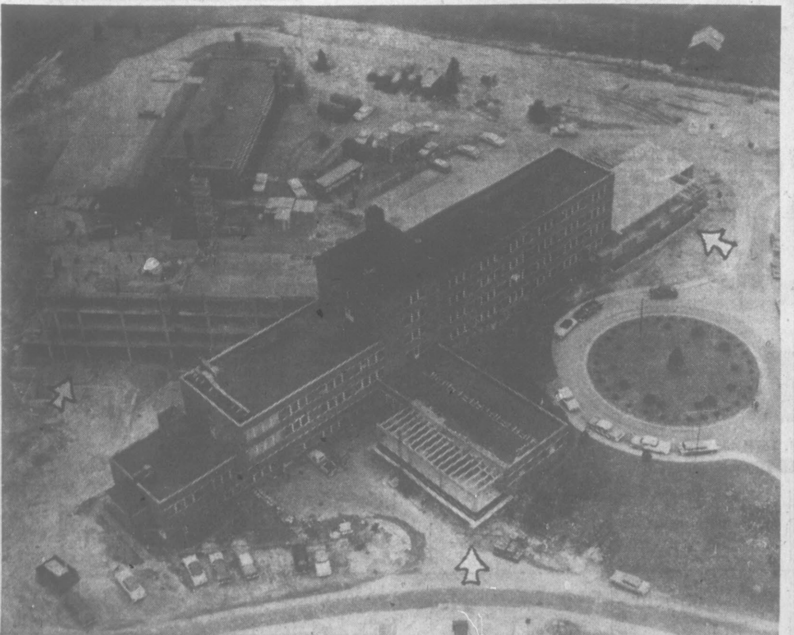
PITT'S LARGEST JOB . . . for 1959 was beginning $1.7 million addition to Pitt Memorial Hospital in suburban Greenville. Arrows indicate three additions. (Reflector staff photo — flown by Greenville Air Service.)
