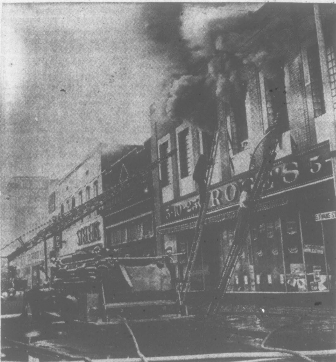
ROSE'S FIRE —Damage amounted to a quarter of a million dollars when Rose's Variety Store was hit by fire on Aug. 28. The blaze began in the second floor of the building. Renovation of the burned structure is now underway.
