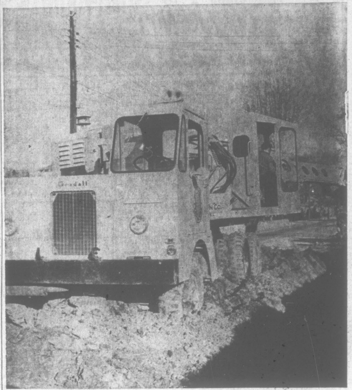
HIGHWAY WORK IN BETHEL —Storm drainage is being installed along U. S. 64 in Bethel in preparation for placing curb and gutter along the highway. The State Highway Commission recently awarded the contract for installation of curb and gutter on U. S. 64 in Bethel. Reflector Staff Photo).
