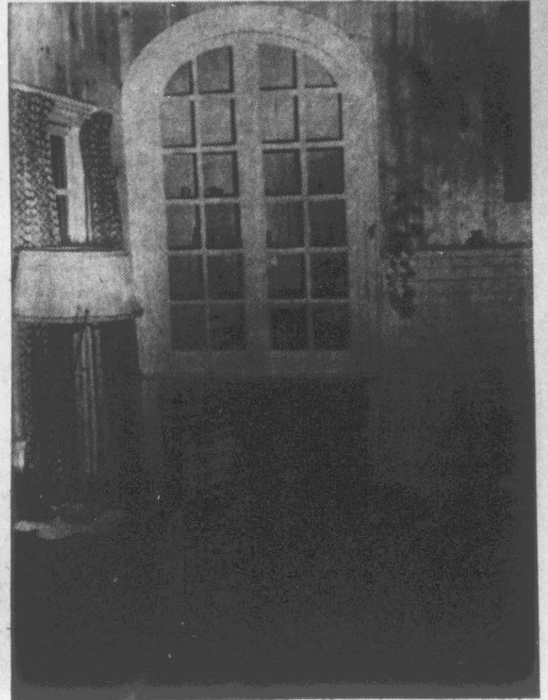
INTERIOR . . . of 200-year-old house has been partially restored by owner, Sam McLawhorn, Jr., of Grifton.
