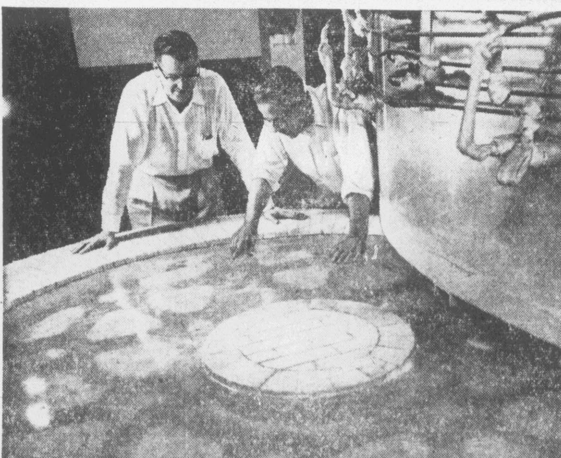
5. Cooling of disk lasted seven months. Engineers examine it before removal starts. Regulated cool-down prevents breakage and eliminates internal stress in glass.
