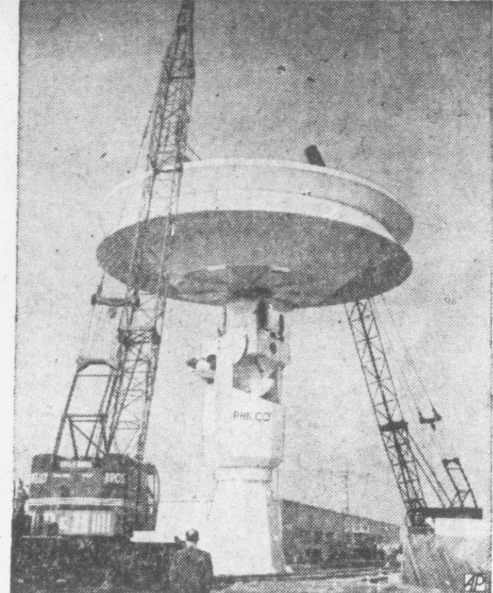
MOVABLE LISTENER — Sixty-foot reflector antenna is set up at Palo Alto, Calif. The satellite-tracking antenna will have movement in three directions.
