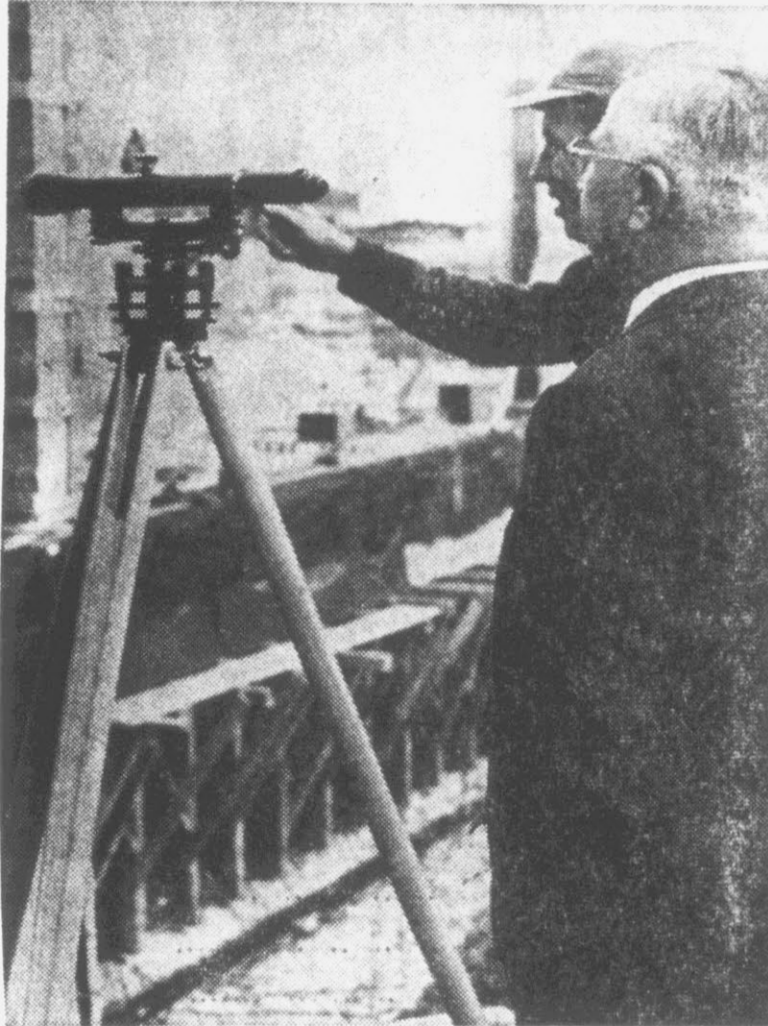
LOOKING OVER . . . site of new three-story wing addition.
