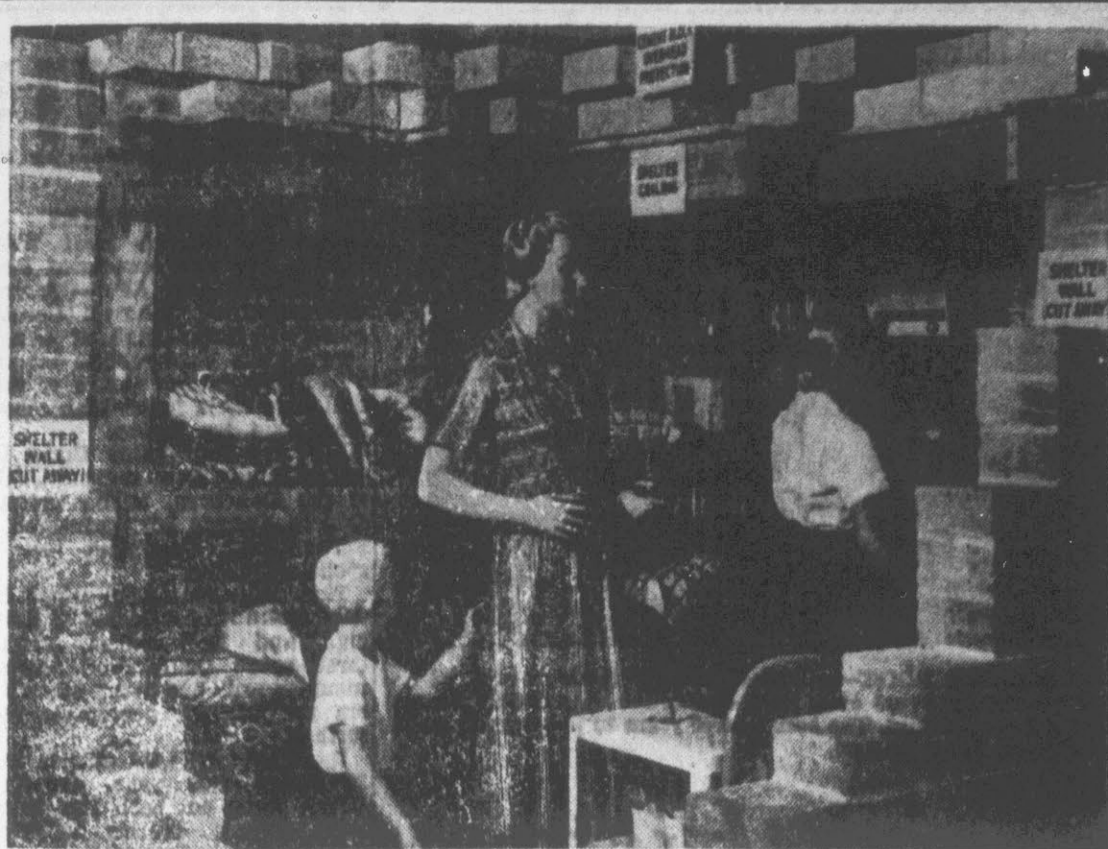
MODEL FALLOUT shelter of concrete blocks shows some of the equipment, supplies and living facilities that would be needed to remain under cover for up to 14 days. This is a basement type shelter adaptable to either rural or suburban homes. The 8-inch solid concrete block walls shown would give the same fallout protection as 12 inches of earth. Details on how to build and equip such a shelter are available by writing Box Home Shelter, Battle Creek, Mich. (OCDM Photo)
