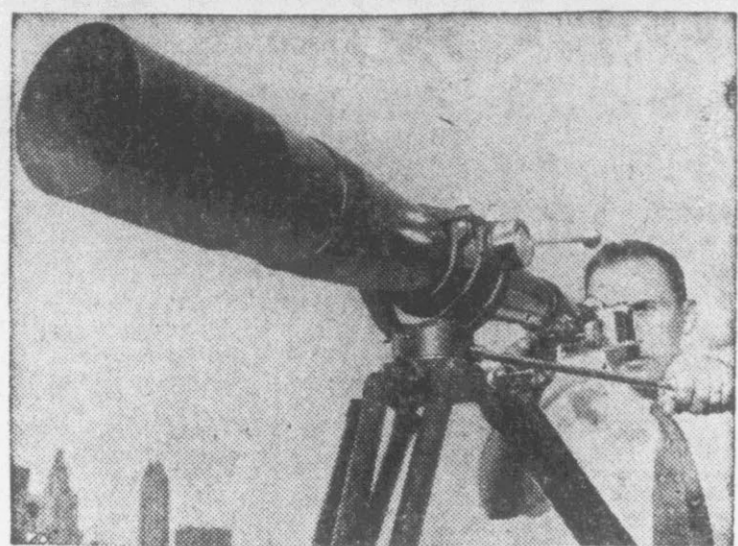
LONG RANGE SHOOTING for close-up results is done with this cannon-like accessory for a single-lens reflex—the 1,000mm telephoto lens for the new Heiland-Pentax H2 35mm camera. Weighing 16 pounds, it comes with its own 30 pound tripod. The camera weighs only 27 ounces.
