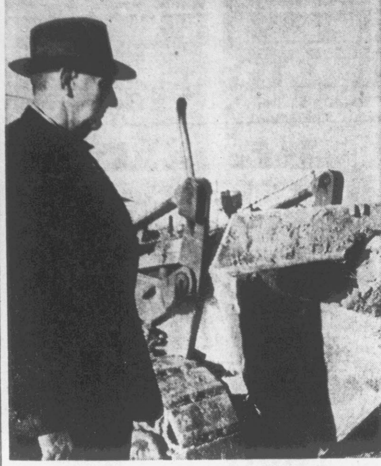
SUPERVISING . . . the removal of dirt on a paving project.
