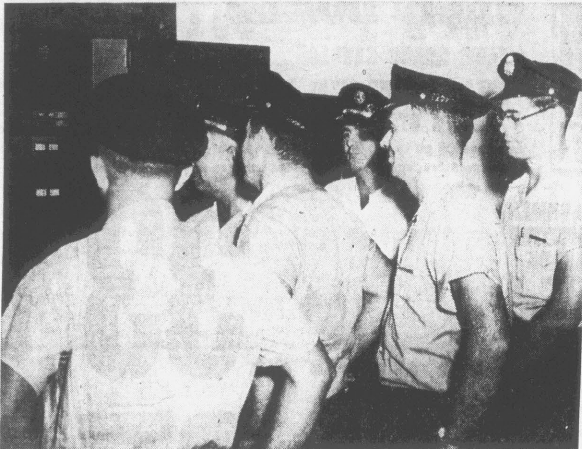
FIRE PREVENTION WEEK INSPECTION —Greenville firemen are shown inspecting a fuse box at Third Street School as a part of their tour of Greenville schools and businesses this week. The firemen tour different buildings in town in order to familiarize themselves with the floor plan of the structures so, in the event of a fire in the building, they will know what to look for. (Reflector Staff Photo)
