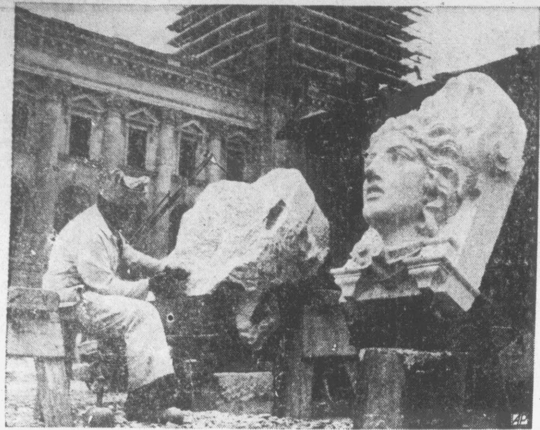
REICHSTAG TOPPER—Stone mason uses plaster model to work on sculpture which will be mounted on roof of the rebuilt Reichstag, background, in Berlin. The historic structure was burned by the Nazis in 1933 and bombed during the last war.
