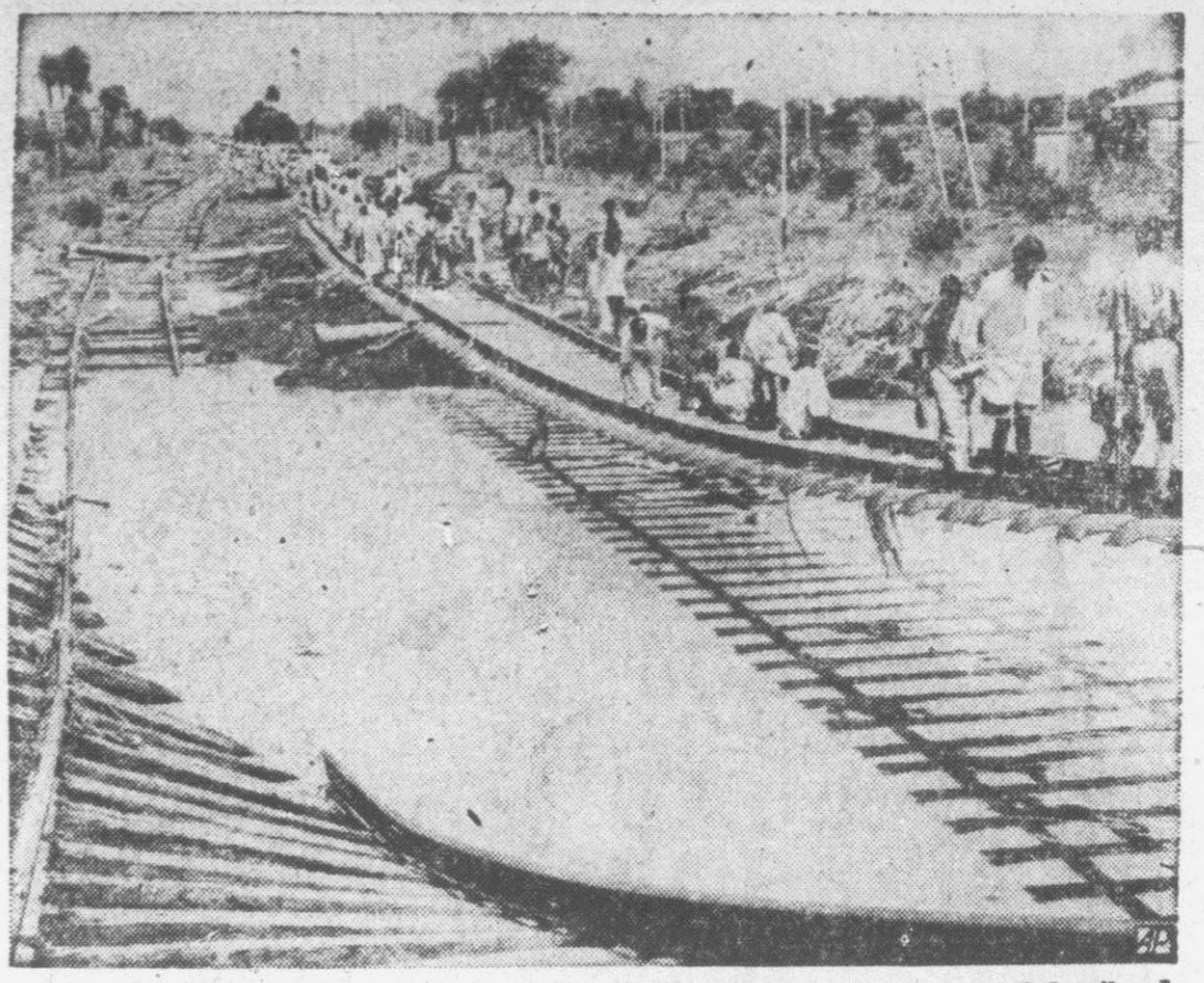
THE RAINS CAME — Refugees pick their way across suspended railroad ties over the Tapi river after monsoon floods swept away bridges in western India. River burst through ancient protecting wall, sweeping away estimated 5,000 dwellings.
