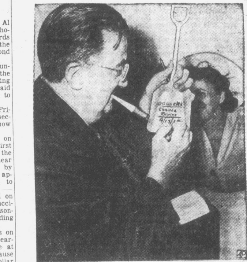
PLEASANT CHORE — Los Angeles Dodgers president Walter O'Malley autographs small shovel as a memento of ground-breaking for Chavez Ravine stadium.
