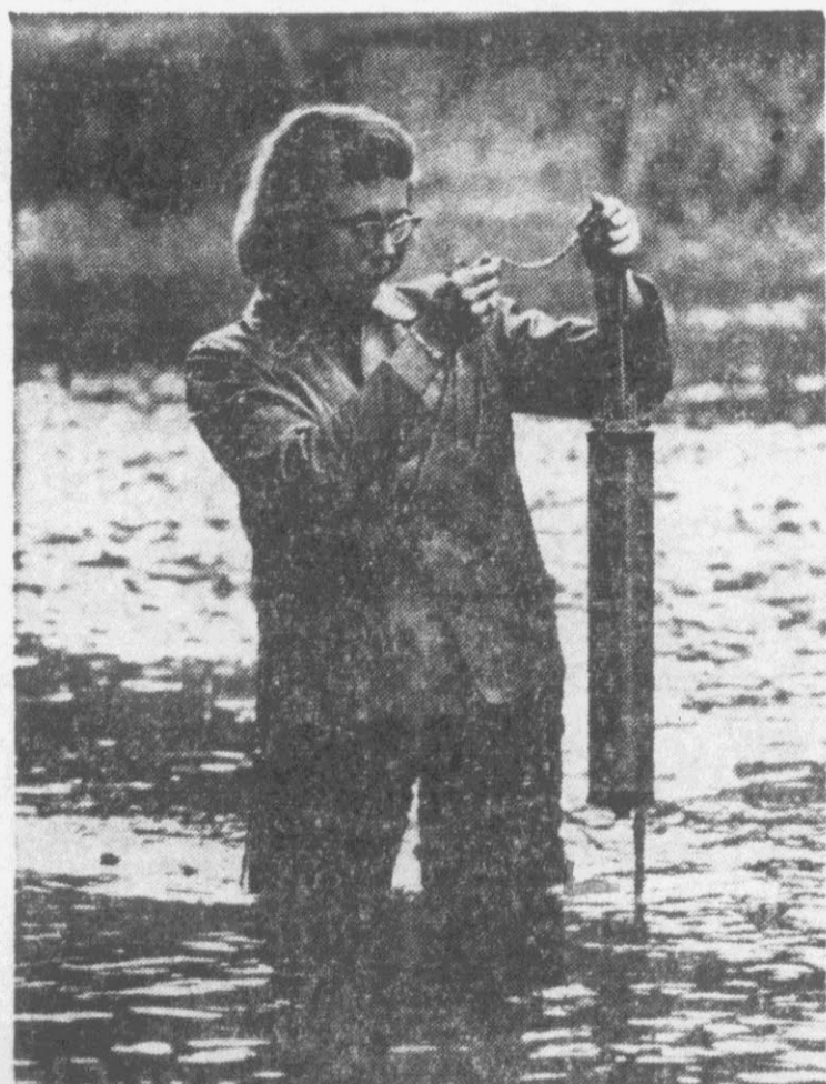
Water is collected with use of big brass cylinder. It's then analyzed for its oxygen content.
