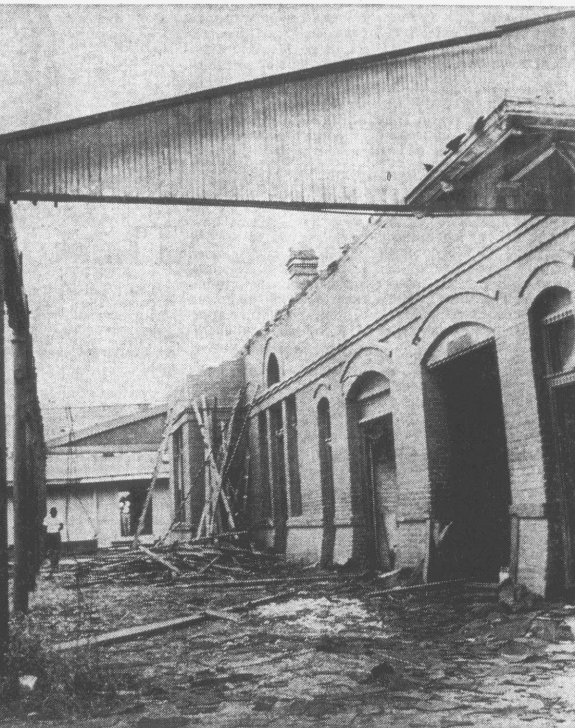
OLD LANDMARK . . . the Norfolk and Southern Passenger Depot on Dickinson Ave. is being torn down to make room for a new brick store building. The property was bought two years ago from the railroad by a fertilizer company and spokesmen for the firm said the new building would be leased. The old passenger station was constructed on the site in 1907 on land which was purchased one year before, and passenger service to Greenville was started that year. The station served Greenville until passenger service was discontinued by the line at the close of business January 1, 1948. The railroad later closed its freight office on Dickinson Ave. and constructed a station just off 14th St. last year. (Reflector Staff Photo)
