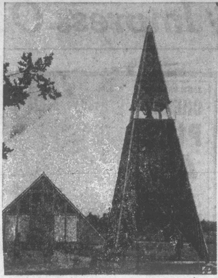
SPATIAL TOWER — It's not a rocket ready to roar into space but the tower of a new church at Gross-Velstedt, Germany. It's wood covered with plastic plates.
