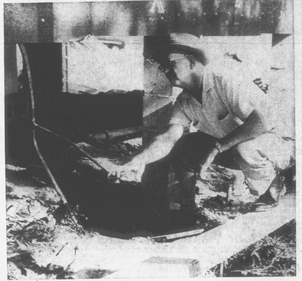
PLUMBING INSPECTION . . . city ordinances provide for proper installation.
