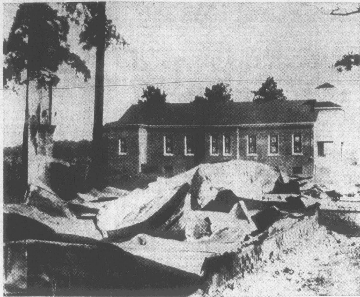
WARREN CHAPEL SCHOOL . . . destroyed by fire early this morning.
