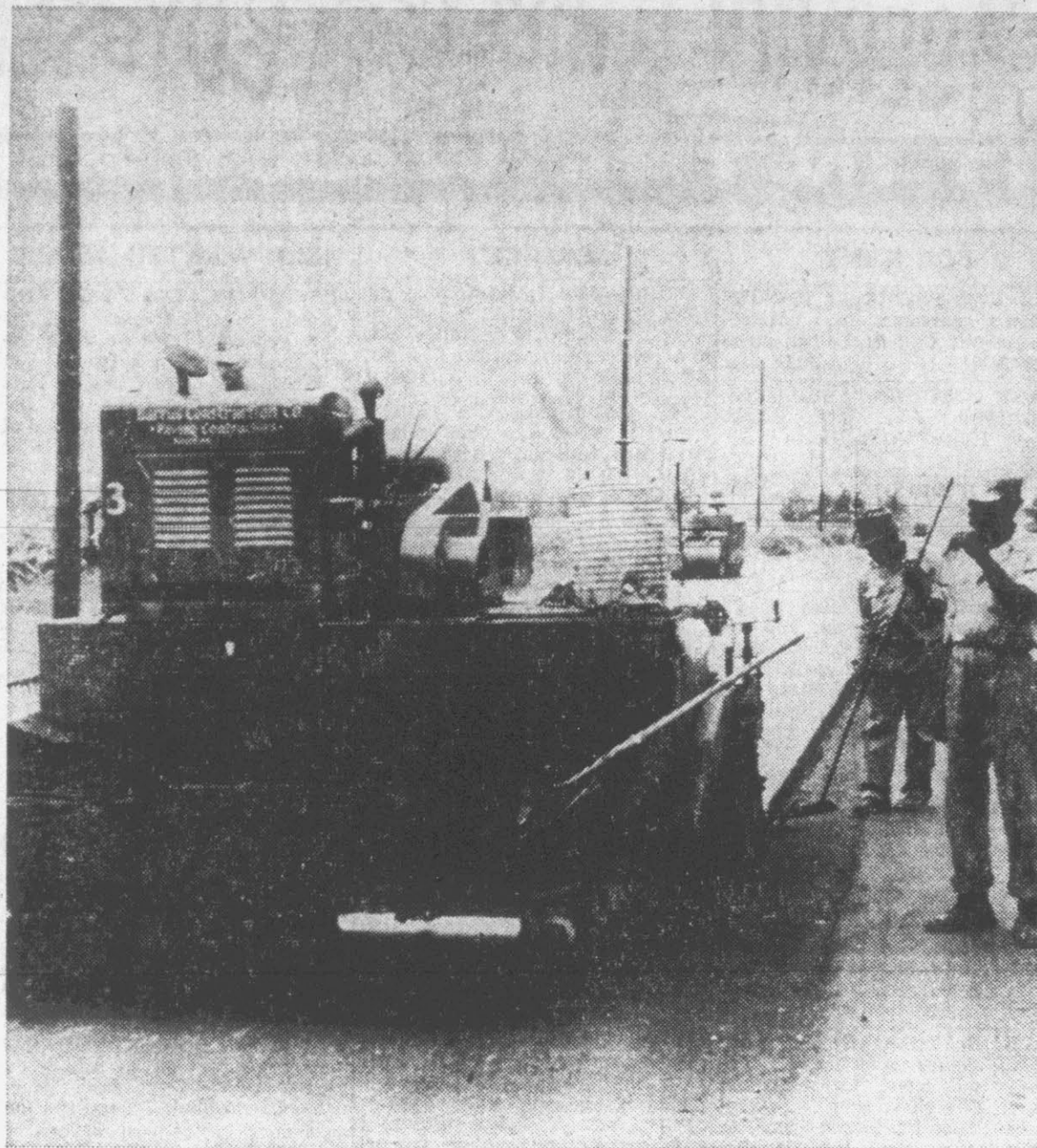
300-DEGREE ASPHALT . . . goes onto the new 60-foot-wide stretch of highway between West End Circle and the South "11" drive-in theater. Workmen here follow the paving machine.
