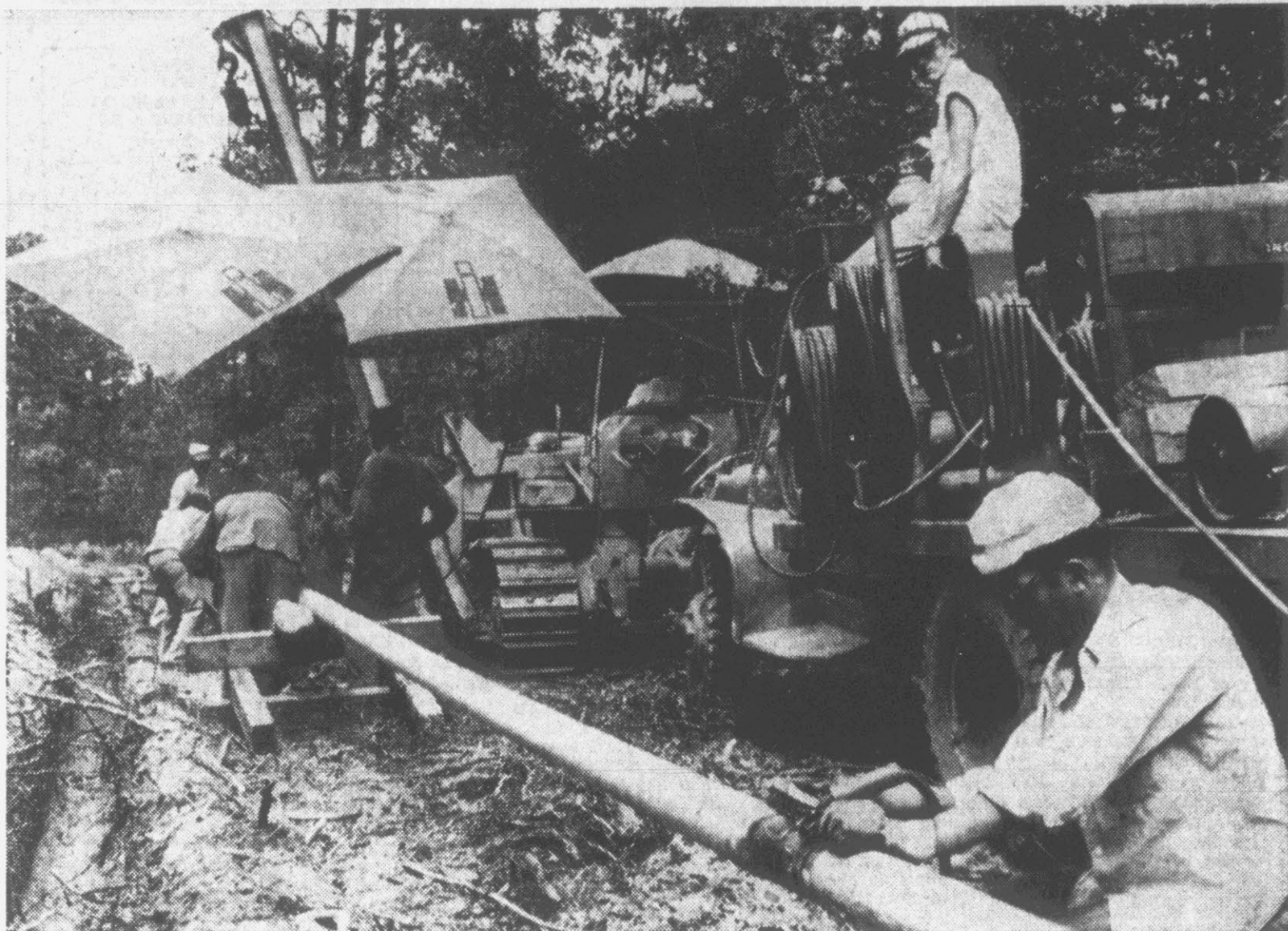
WELDER . . . joints the pipe together as a tracked pipelayer holds the line in place.
