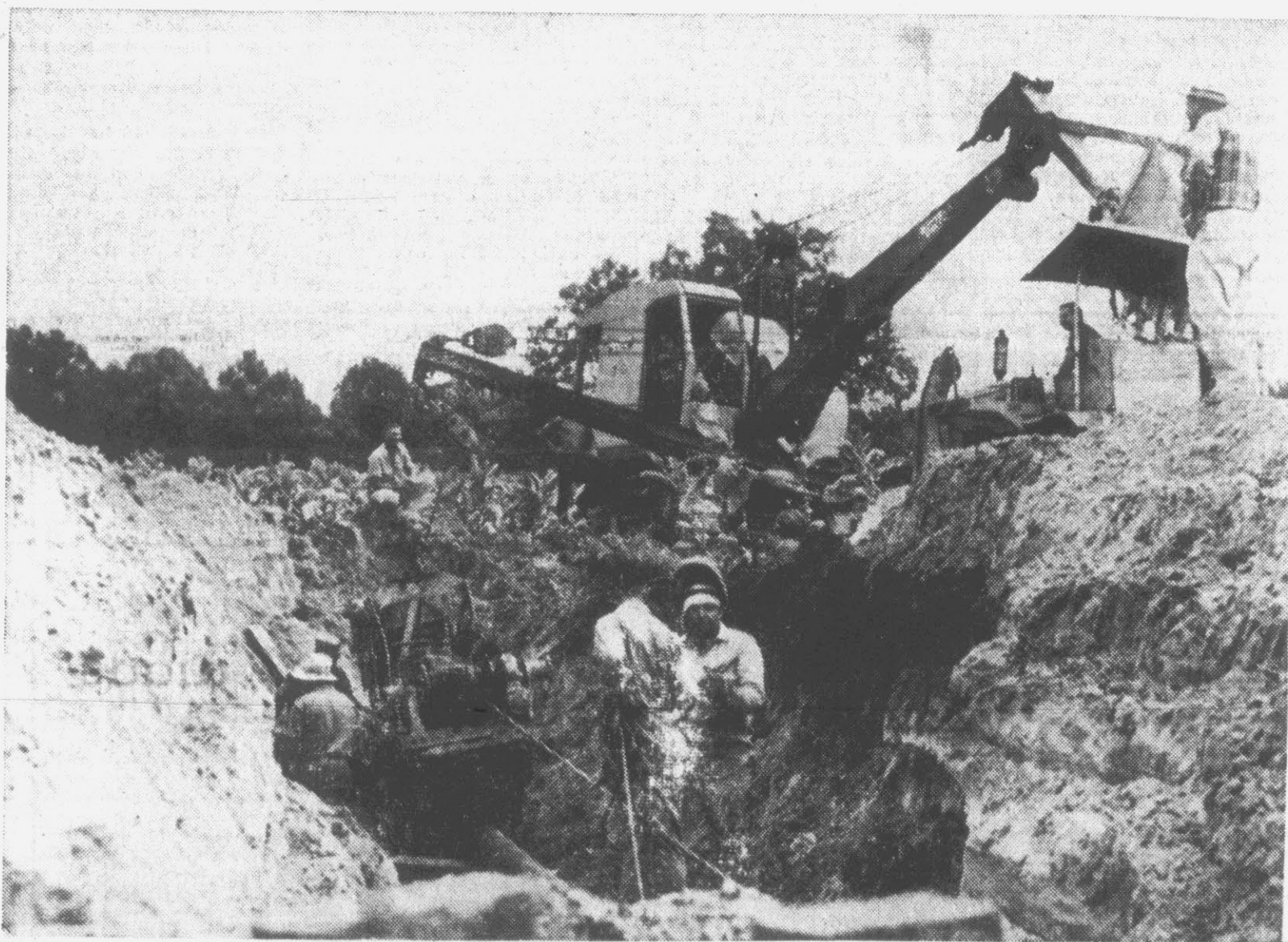
WORKMEN . . . prepare machine which will bore a hole for placement of a six-inch pipe under a highway.
