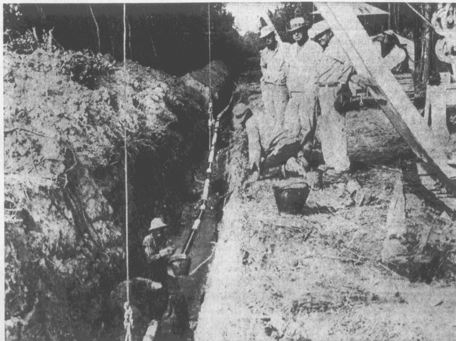
INSPECTORS . . . look on as workmen put finishing touches on a section of line prior to its being covered with dirt
