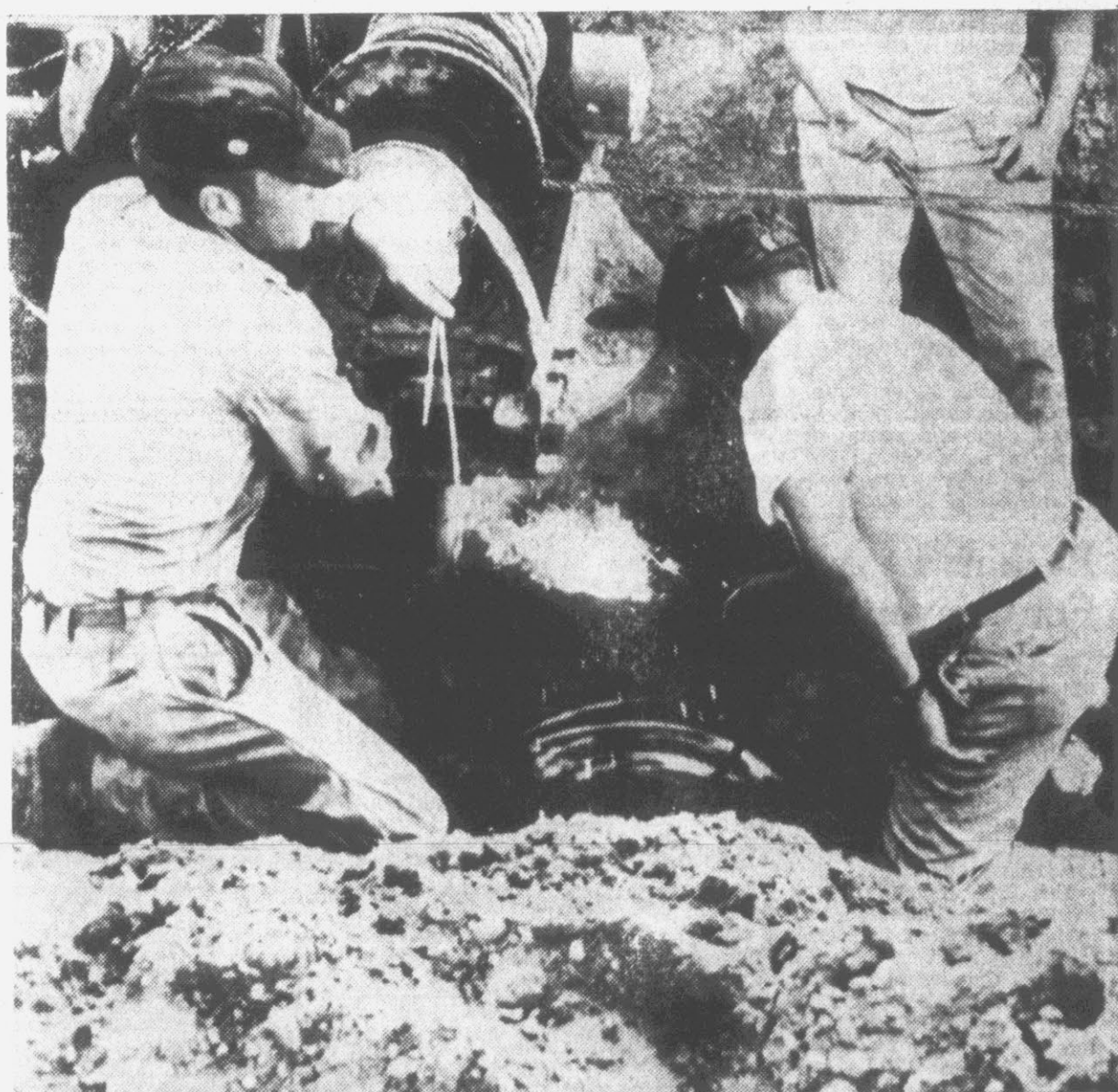
"SPREADMAN" . . . Leverne Curtis, Manager of Gentry's Eastern Division, puts finishing touches on a road crossing with an electric welding unit.
