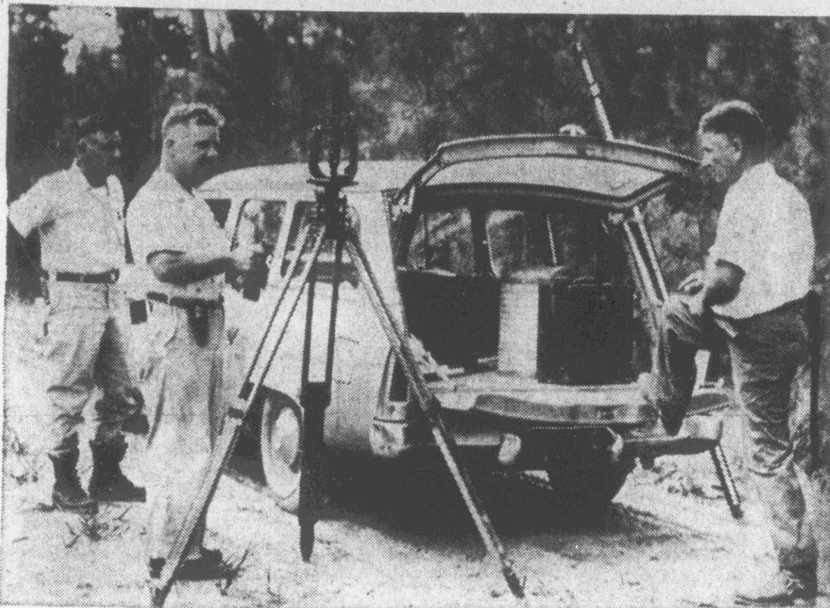
SURVEY TEAM . . . Supervisor Leamon, Engineer Paul McKenna and helper Claude Barrow prepare to survey a line at the Pactolus site of the Voice.
