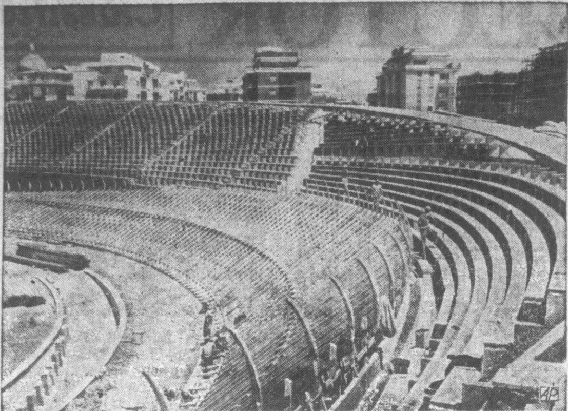
SUMMER CURVE —Foundations for turn are completed in 10,000-seat velodrome under construction in Rome, Italy. Cycling events of 1960 Olympics will utilize track.
