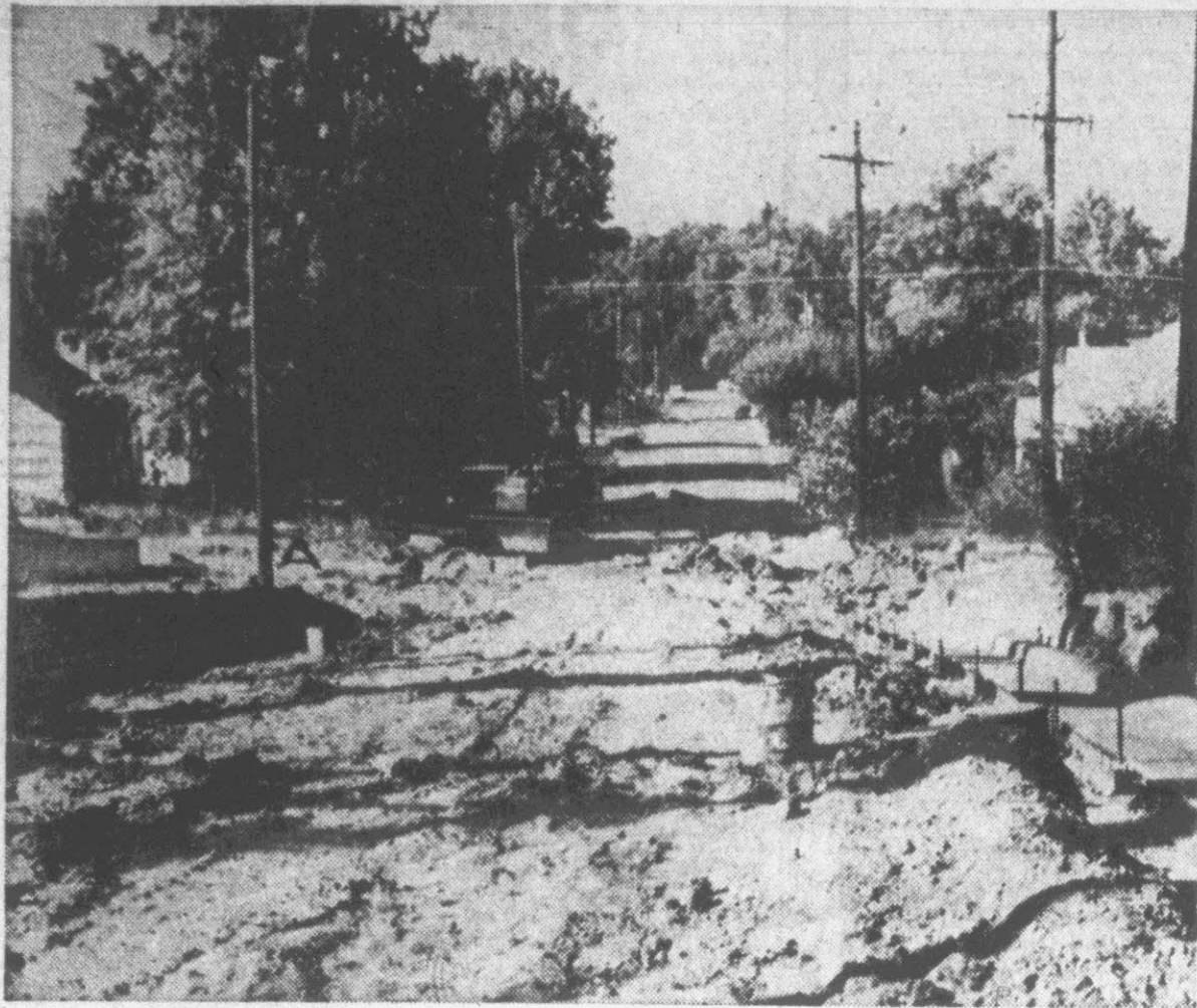
WORK AT JARVIS AND FIRST ST. . . intersection being tied in with First St. cross town route.
