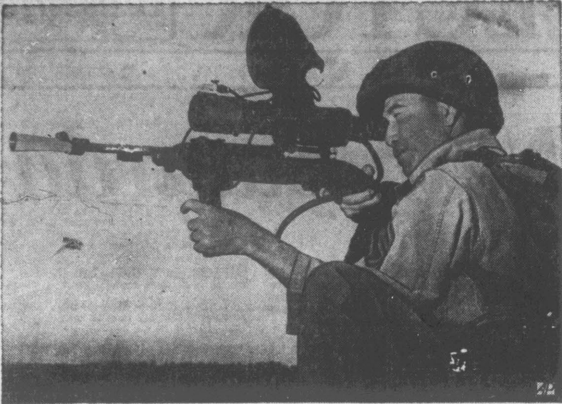
NIGHT SIGHT — Soldier tests T-1 infrared sight on carbine at Fort Benning, Ga., infantry school. Device is used to "see" enemy at night with invisible infrared rays.
