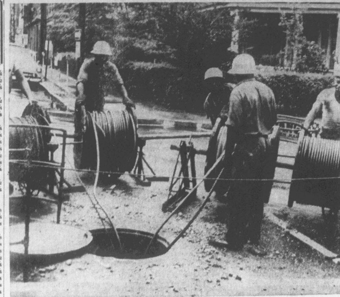
LAYING CABLE — Utilities crews yesterday were feeding cable into an open manhole to be forced underground to the recently completed transformer vault on Fifth St. The transformer will be installed within the next few weeks.
