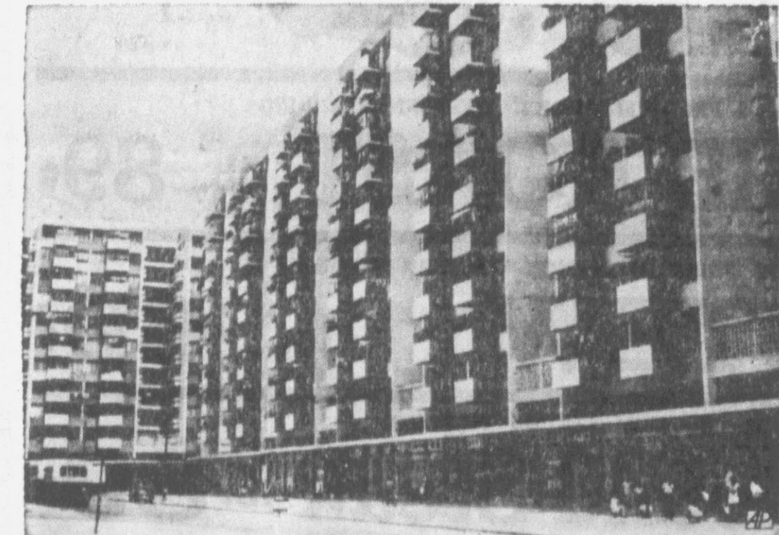
REFUGE FROM REDS—This is one of the many apartment building projects that Hong Kong has erected to house hundreds of thousands of refugees from Red China.
