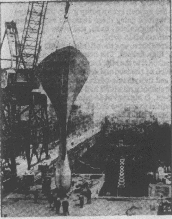
SHAPING UP—The 56-foot-high bow is moved into position for welding to the nuclear-powered cruiser, U.S.S. Long Beach, under construction at Quincy, Mass.
