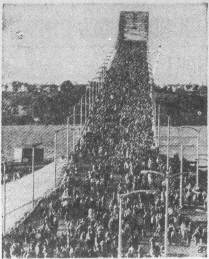
SPAN-STROLLERS — Part of crowd of 100,000 pedestrians walks across new harbor bridge in Auckland, N. Z., prior to official opening as a vehicular crossing.
