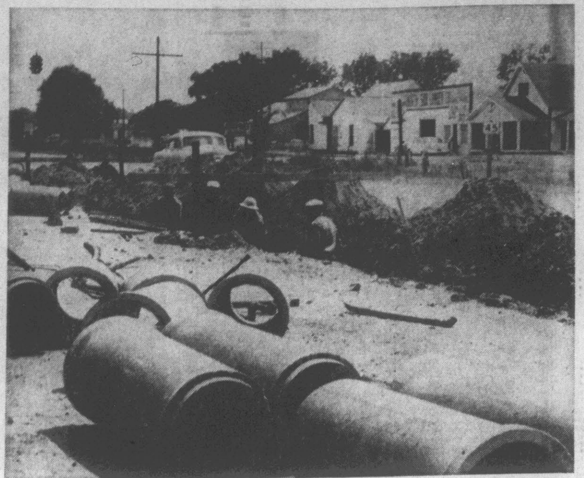
STORM DRAIN INSTALLATION . . . Workmen are installing storm drains on North Greene St. prior to laying curb and gutter on the road. Construction on the State Highway Commission project began last week.
