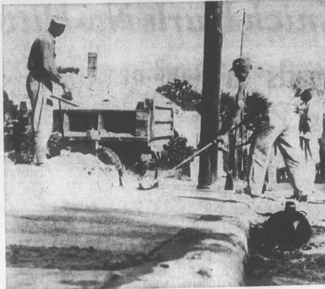
SIDEWALK INSTALLED —A sidewalk is being installed by the city along the block on the northeast side of the Dickinson Ave. and 14th St. intersection. The northeast corner is also being cut back to allow better movement of traffic at the offset intersection. (Reflector Staff Photo)
