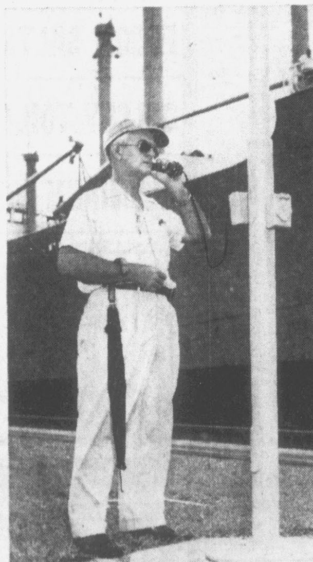
Lockmaster Richard Abel, on lock wall, phones an order to the Miraflores Locks control tower. . . and, in tower, Frank Dolan, control house operator, throws small switch to swing open the 750-ton gate leaves.
