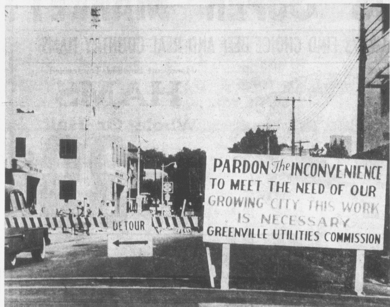
DETOUR FOR PROGRESS —Greenville Utilities apologizes to detouring motorists by means of this sign erected at Fifth and Washington Sts. Fifth St. between Washington and Greene has been closed to traffic while utilities employees make electrical installations under the street. An underground transformer vault, manhole and underground electrical cable are included in the project. Superintendent Leonard Bloxam said that Washington St. between Fifth and Dickinson Ave. will be closed for a short time in connection with the project also after Fifth is re-opened to traffic. (Reflector Staff Photo)
