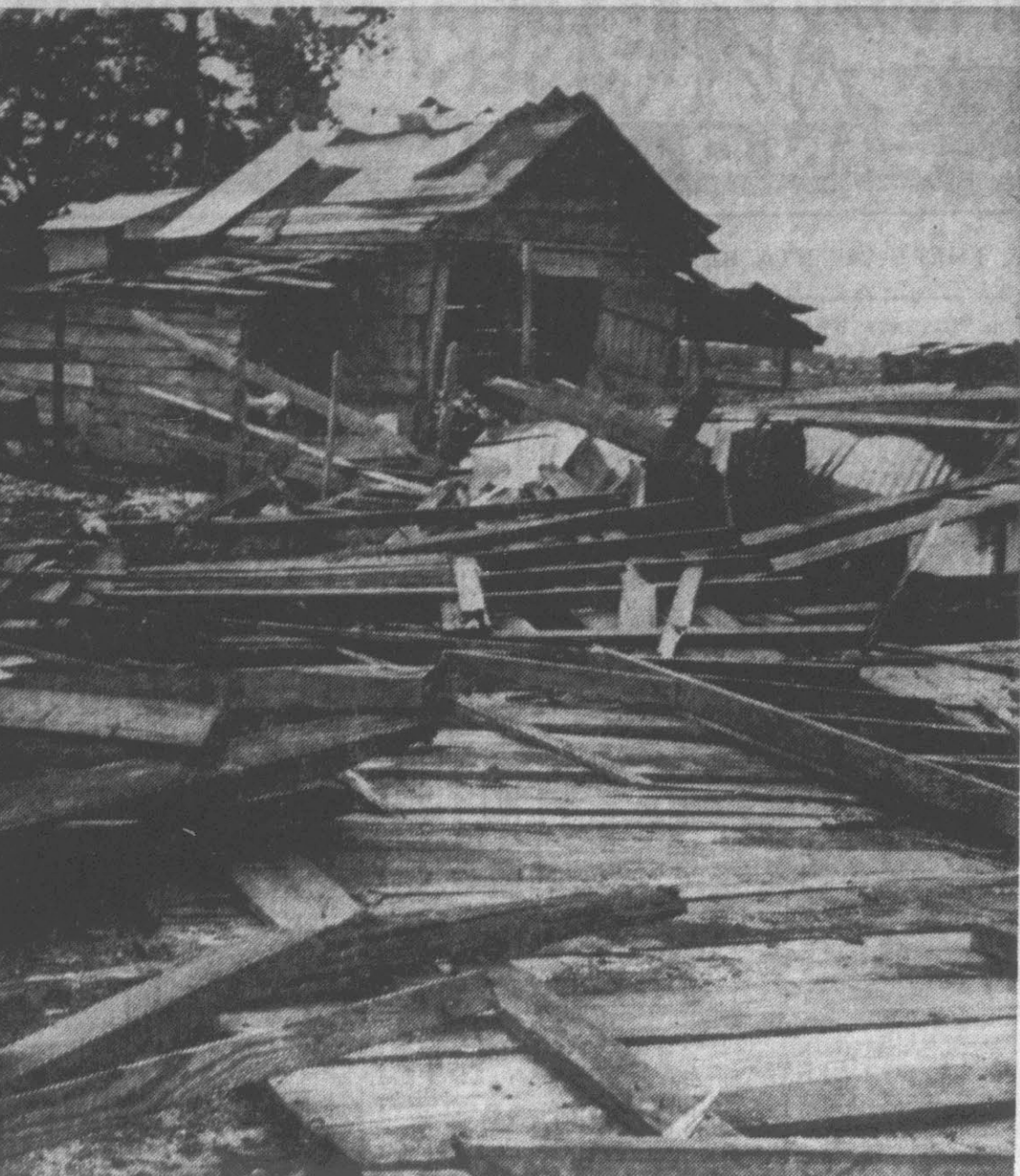
TORNADO DAMAGE . . . Remains of a barn and out-building on the Annie Brown farm near Ayden.
