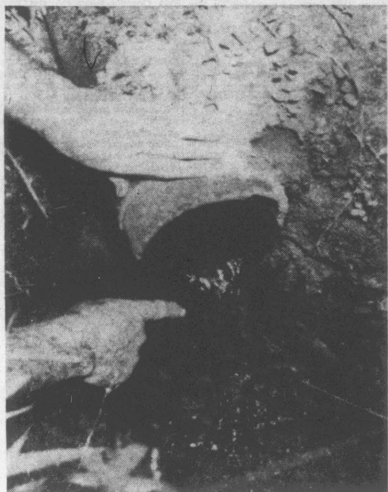
TILE INSTALLED UNDER FIELDS . . . water flows into ditches then to creeks.
