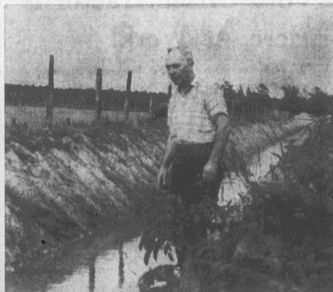
EAGLES LOOKS OVER NEW DRAINAGE DITCH . . . more drainage has increased load on creeks such as Grindle.
