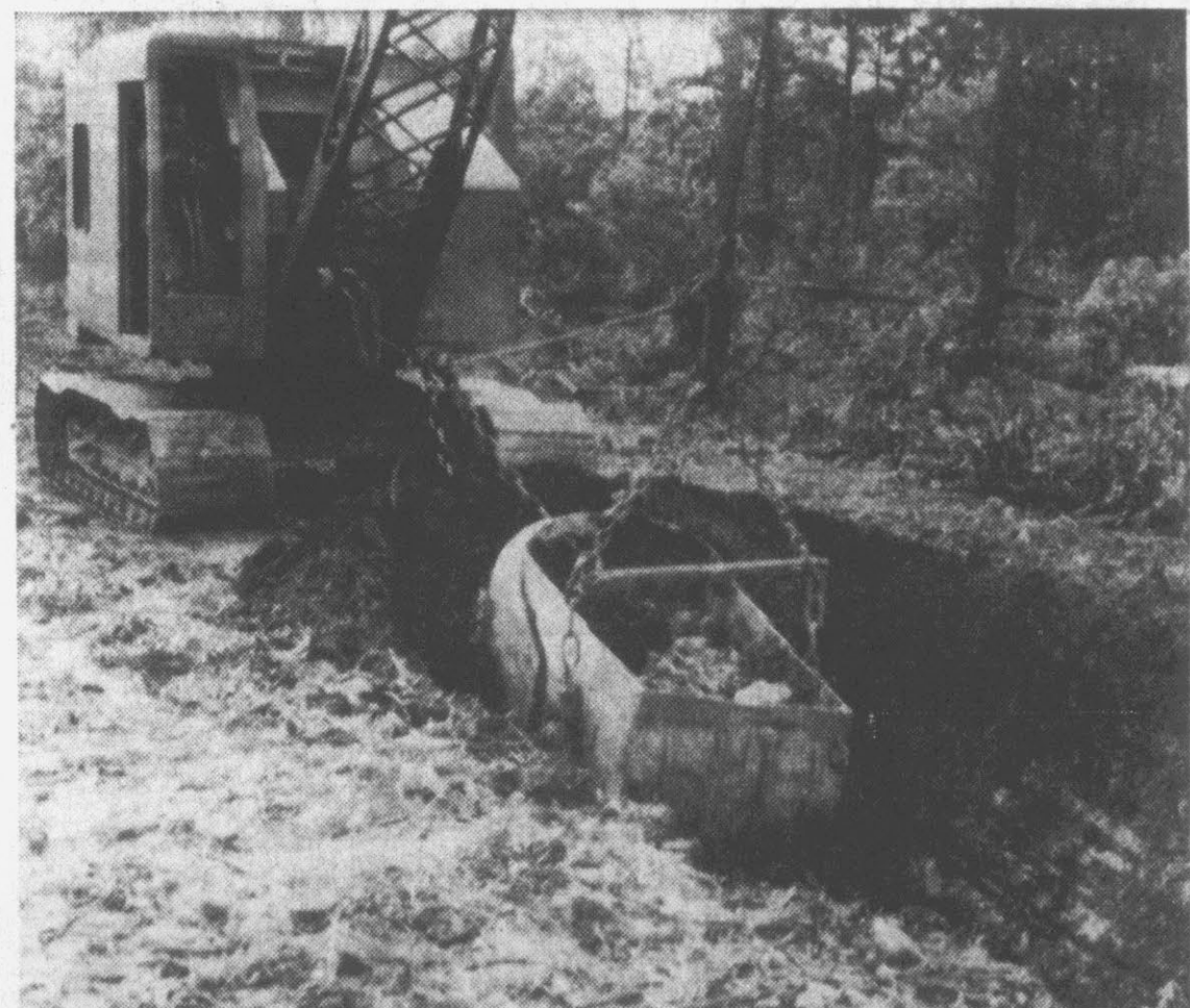
DRAG LINES AT WORK . . . broad canals being dug to drain farm land.
