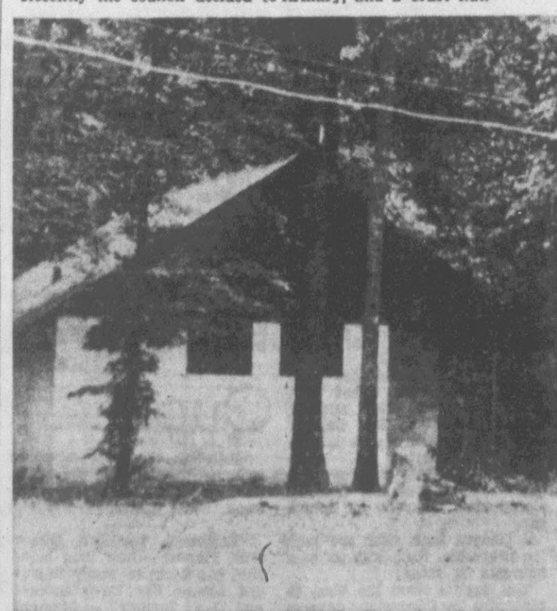
CAMP HARDEE BUILDINGS . . . will have new additions by camp time, June 14.
