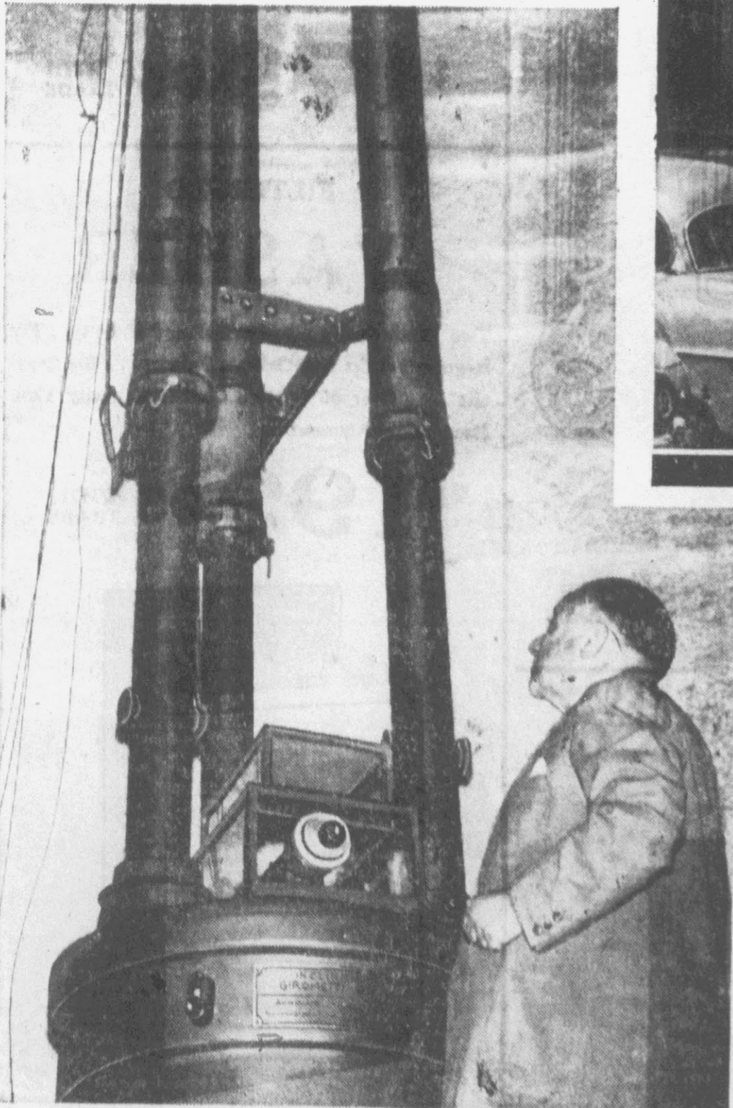
Italian scientist, Prof. Carlo Vallini, studies tower's inclinometer which measures precise degree of tower's constantly changing incline.
