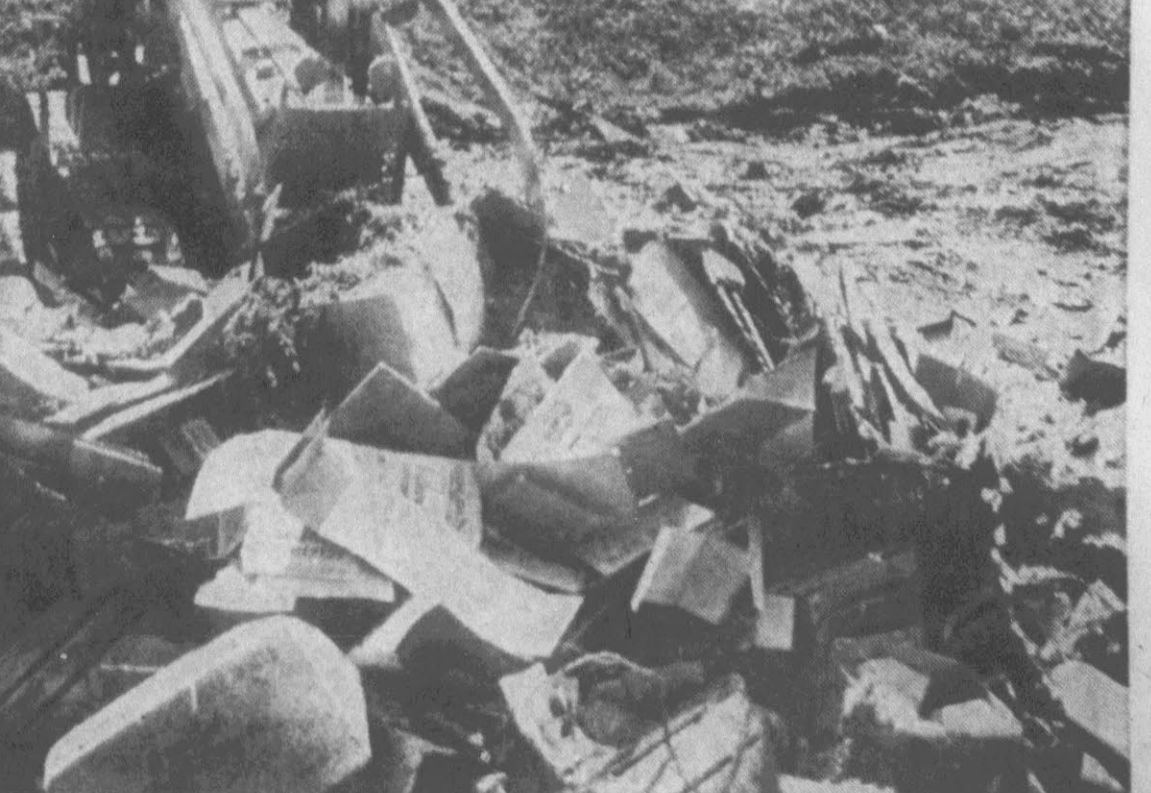
LANDFILL GARBAGE DISPOSAL OPERATION AT FARMVILLE . . . Replaces Open Pit Type Of Garbage Disposal Formerly Used
