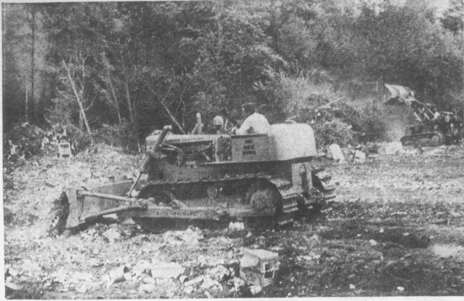
NEW CITY DUMP OPERATION—The city has begun a modified land fill operation at the city dump behind Greenwood Cemetery. This leased tractor is at work daily covering the refuse with dirt. A prisoner-operator is retained to handle the tractor. It is hoped the new method will eliminate fires and rodents at the city dump. (Reflector Staff Photo)
