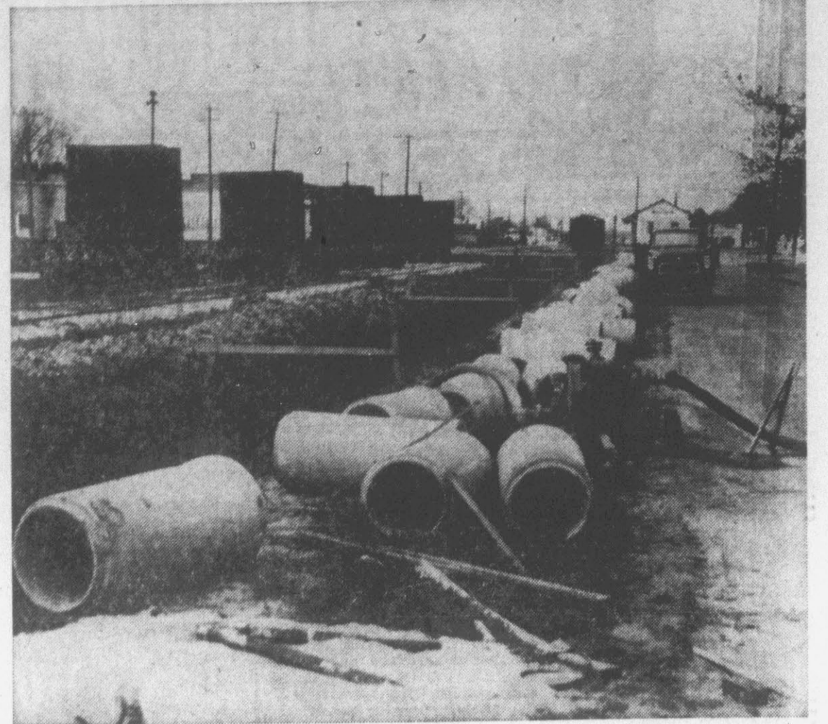
WINTERVILLE DRAINAGE PROJECT . . . will be completed in about two weeks.
