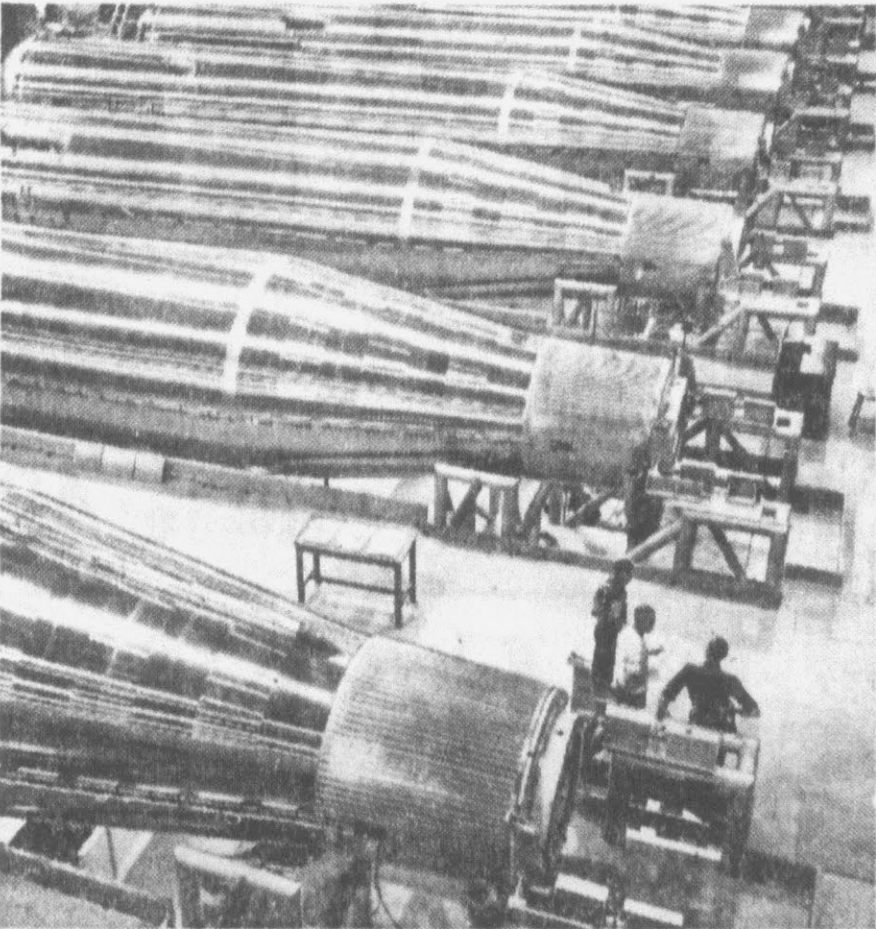
ATLAS intercontinental ballistic missiles are assembled in San Diego, Calif., plant. The stainless steel missile—9 feet in diameter and 80 feet long—has 15,000 mile-per-hour speed.
