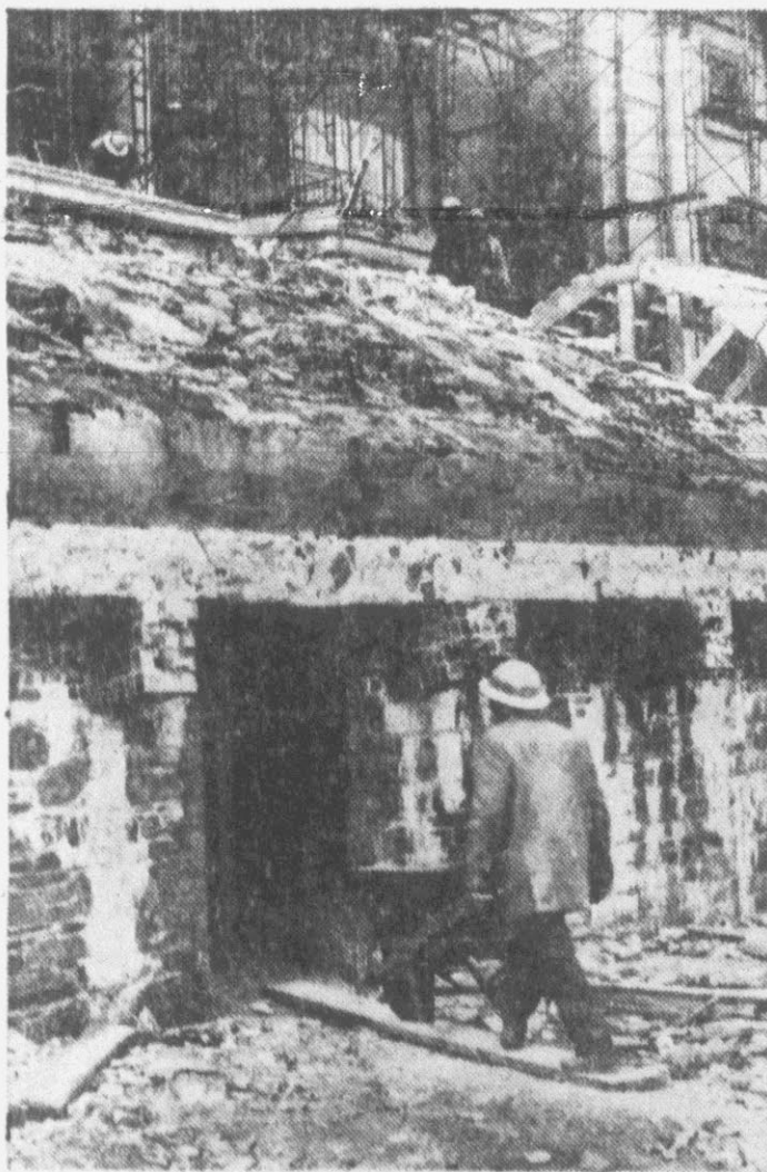
Workman enters passageway to remove debris from space under demolished steps.
