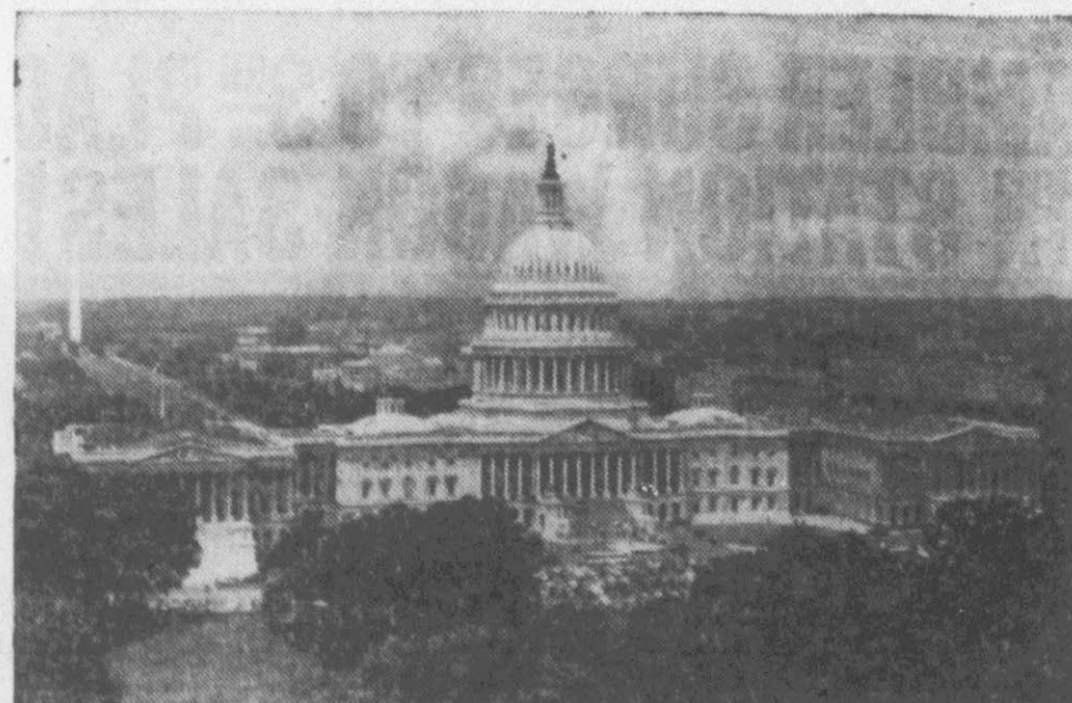
The Capitol as it looked before present remodeling job.
