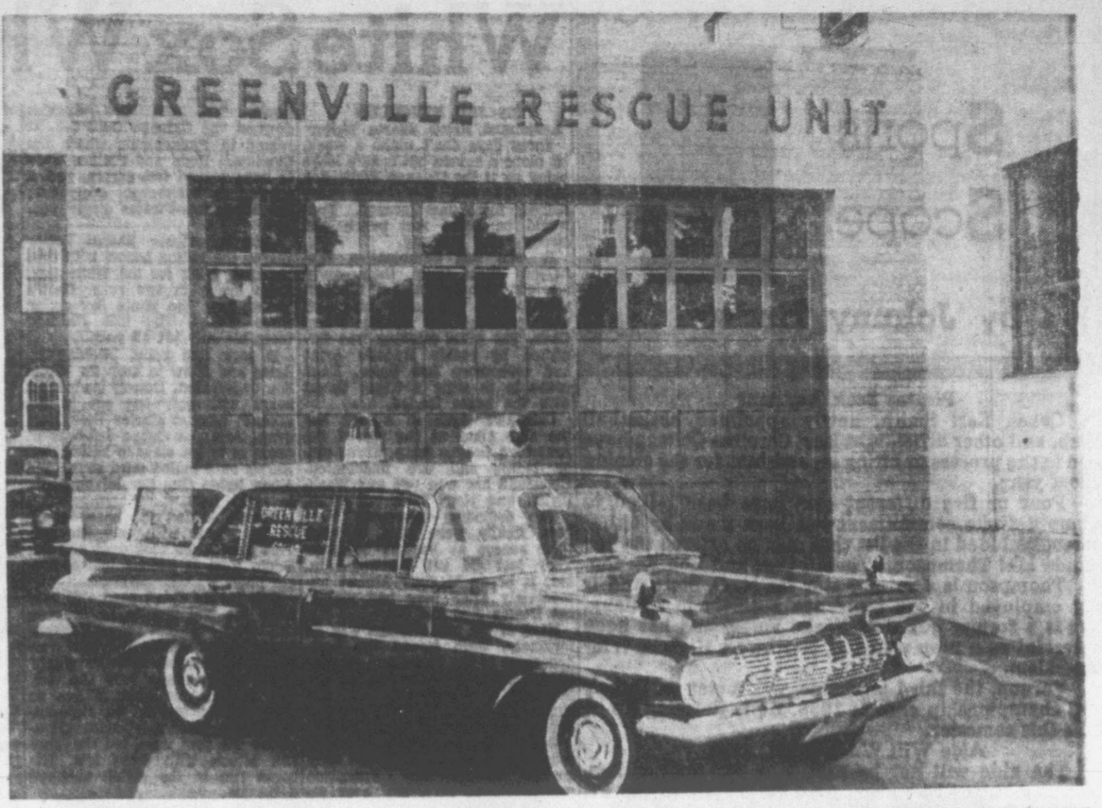
RESCUE BUILDING—Above is the new Greenville Rescue Squad annex to the Central Fire Station. In front is the ambulance which was recently placed in service by the squad. The squad has a second ambulance, purchased 10 years ago; a disaster squad truck; floodlight trailer; two boats for dragging operations, along with other equipment. (Reflector Staff Photo)
