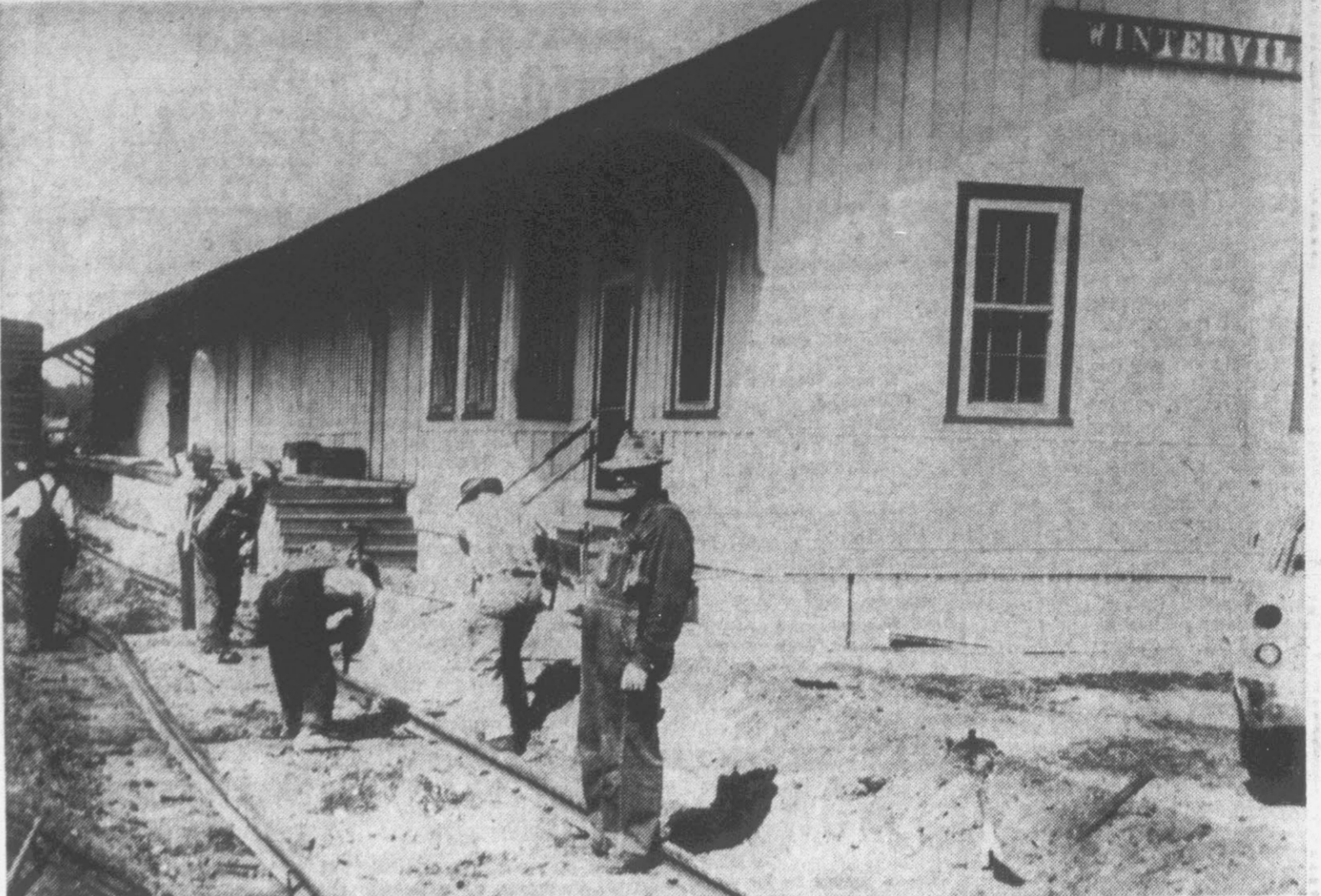
SECTION CREWS AT WORK—A familiar scene along any railroad are the section crews at work. Here, an ACL crew is shown repairing a spur track at the railroad's Winterville depot.
