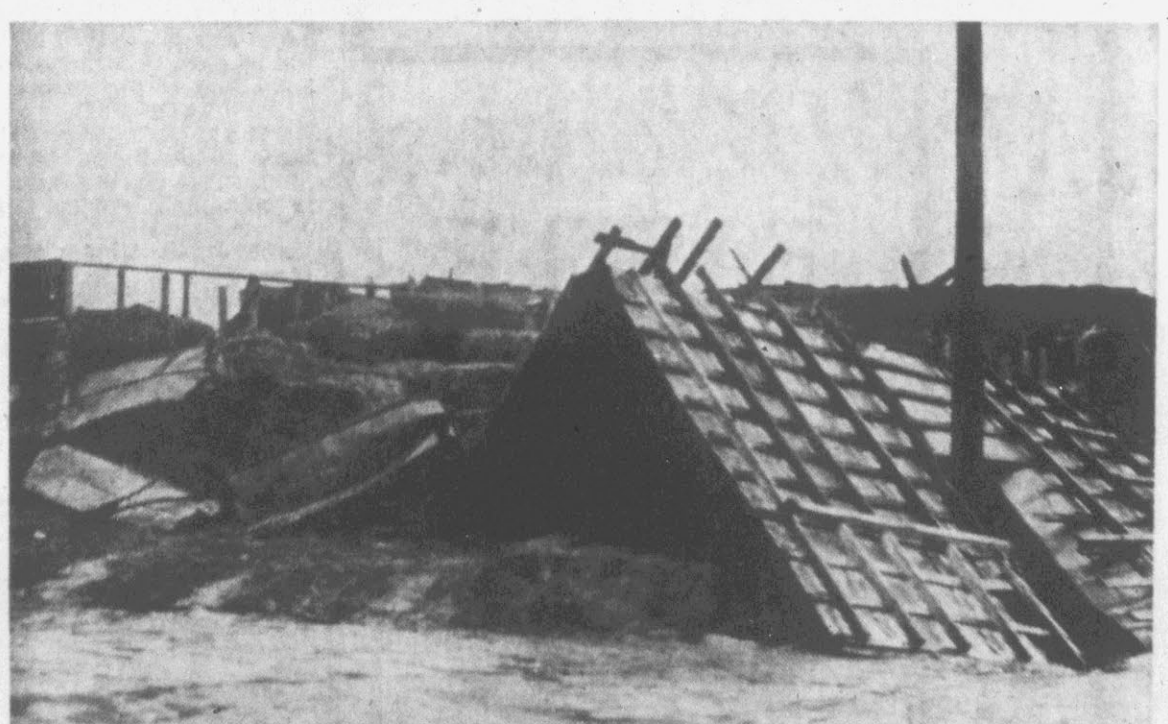
LINE AND MYRTLE AVES. . . Roof of hay barn torn off.
