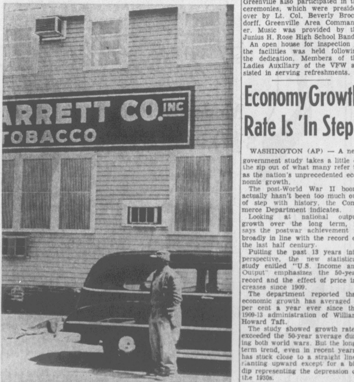
ACCIDENT FATAL FOR WORKER . . . falls from factory roof.
