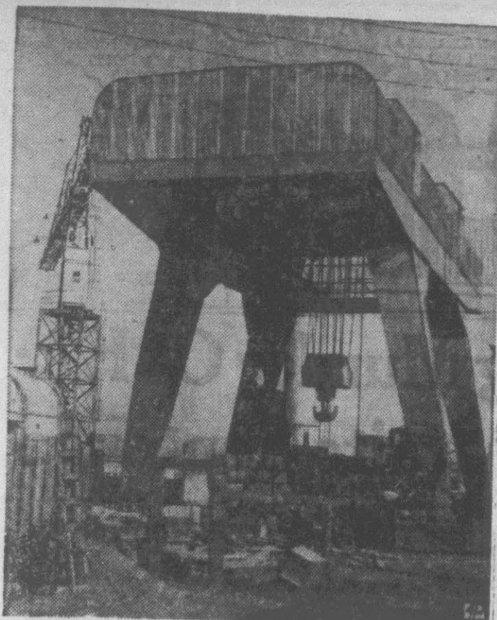
GIANT LIFT — A huge 235-ton crane straddles flood gates of tidal estuary of the Rance river at Saint Malo, France, to lower equipment to harness the tides.
