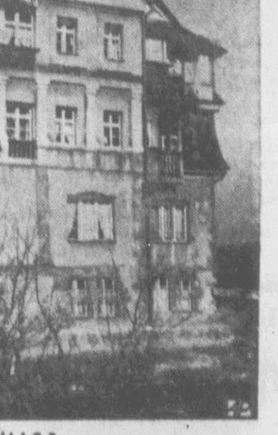
CAN YOU TOP THIS? —Even long-time residents can't say why small house is atop main house in Hagensbuchbach, West Germany. It was built 40 years ago.
