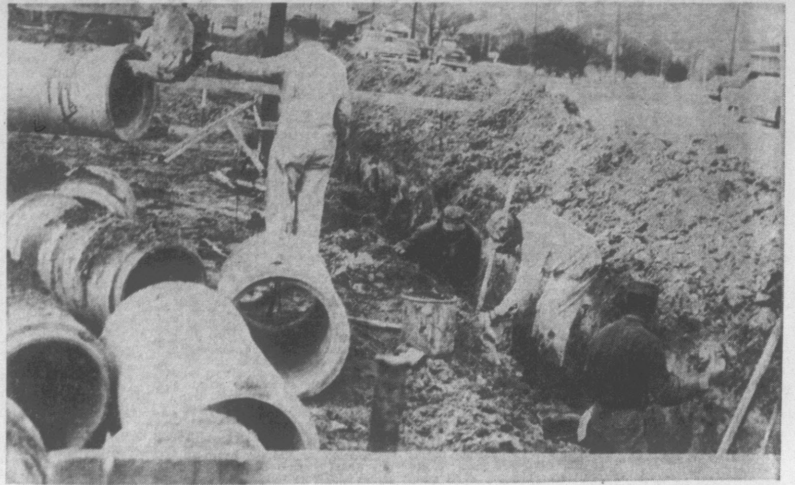
HIGHWAY WORK CONTINUES—Workmen are installing drainage tile on portions of N. C. 11 as part of a project which will result in the highway becoming a four-lane thoroughfare between West End Circle and the South 11 Drive-In Theater. The portion of the expanded highway within the Greenville city limits will have curbs and gutters. (Reflector Staff Photo)
