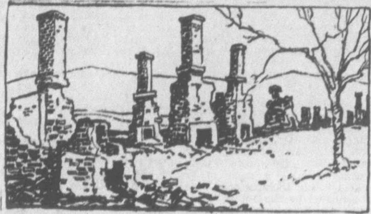
Line of chimneys marks position of barracks at Fort Union, once largest fort in the Southwest.
