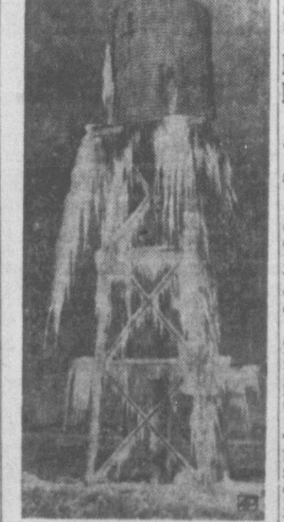
FROZEN DRIP—Water falling from this windmill pump tower froze to form this pretty pattern when sub-freezing temperatures hit area around Dallas, Texas.
