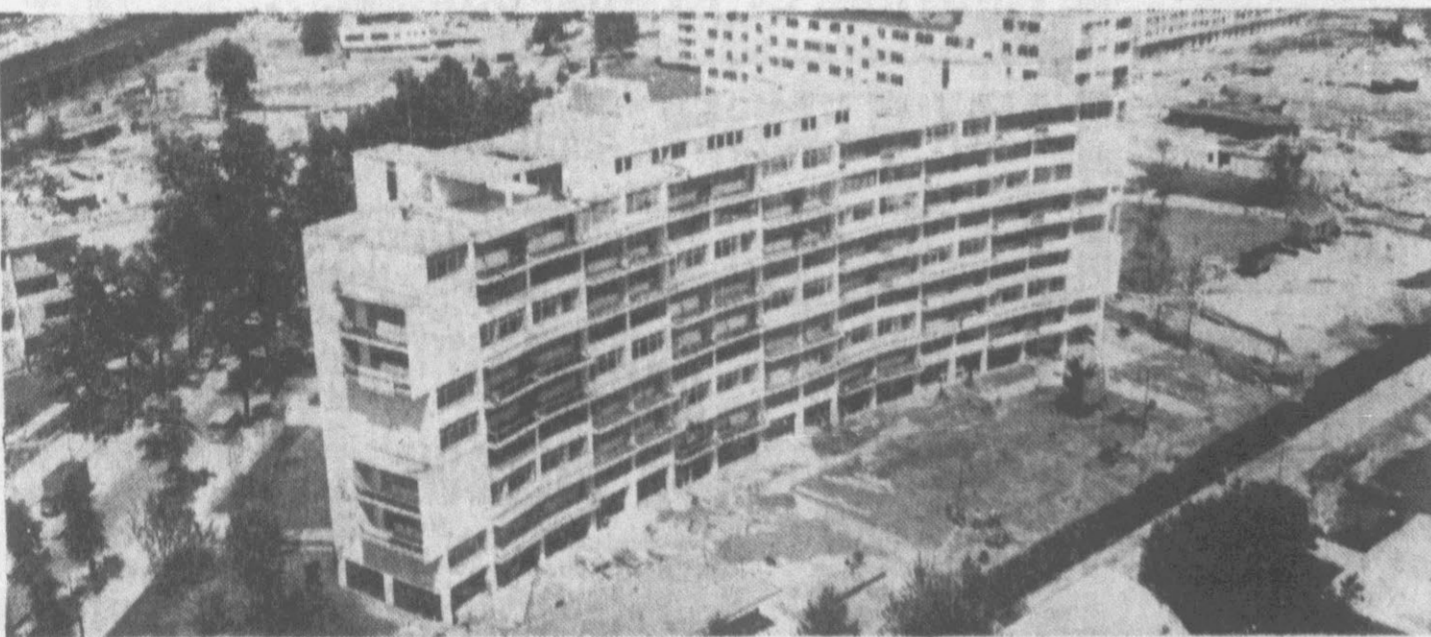
Many modern buildings have risen in recent years to cover the scars of war in West Berlin.
